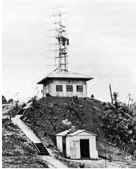
EARLY RADAR INSTALLATION (SCR-271) in Panama.
