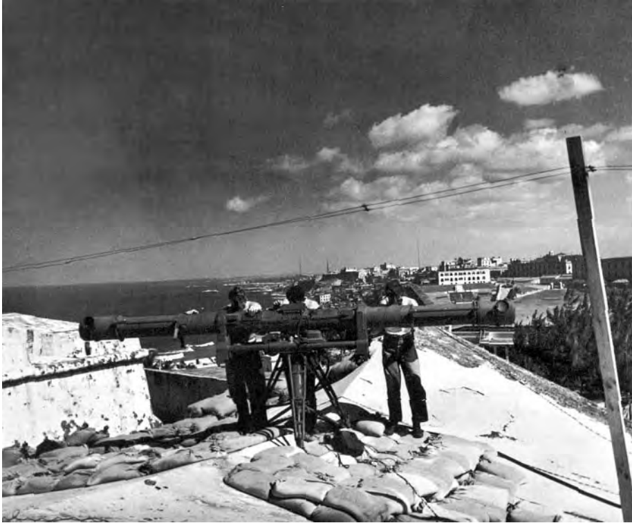
OPTICAL HEIGHT FINDER MOUNTED ON OLD EL MORRO FORTRESS, San Juan, Puerto Rico . U.S. Army post is visible in background.
