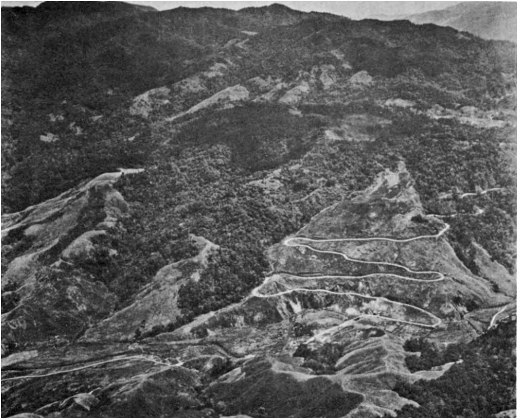
ROUTE 5, winding south from Santa Fe.
