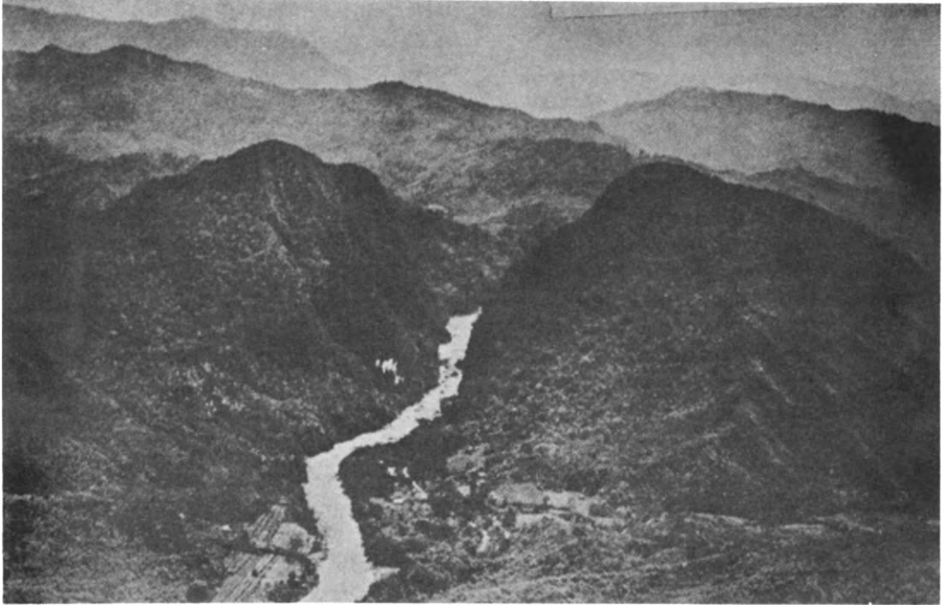
6TH DIVISION APPROACH TO WAWA DAM
