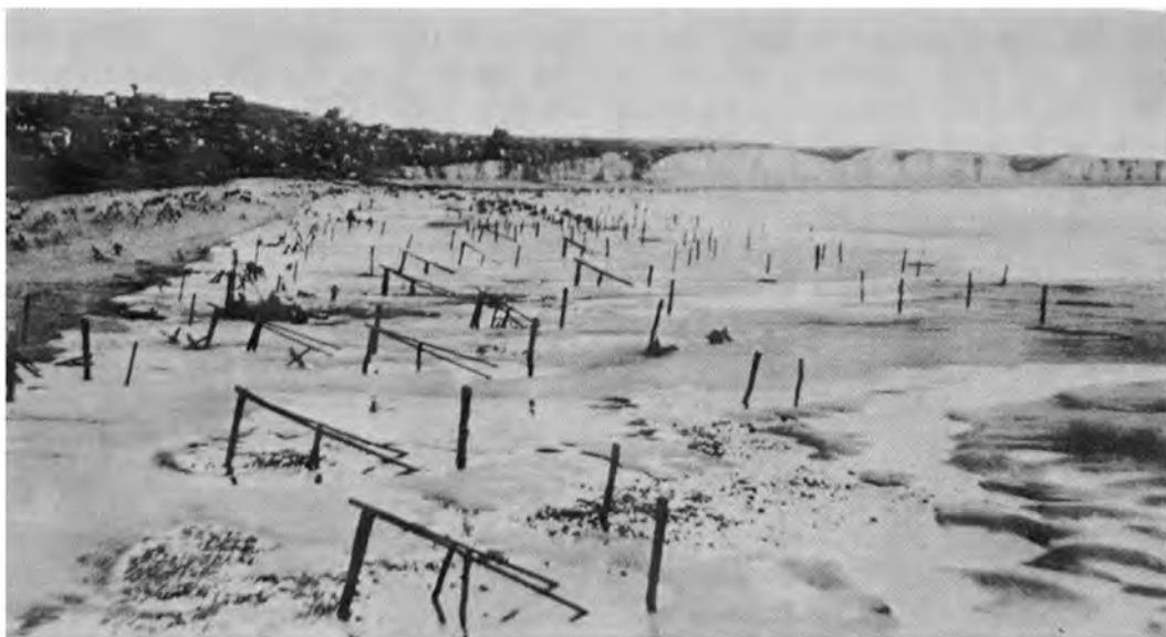
ANTILANDING OBSTACLES under construction on a French beach (above). Lower picture shows Belgian Gate.
