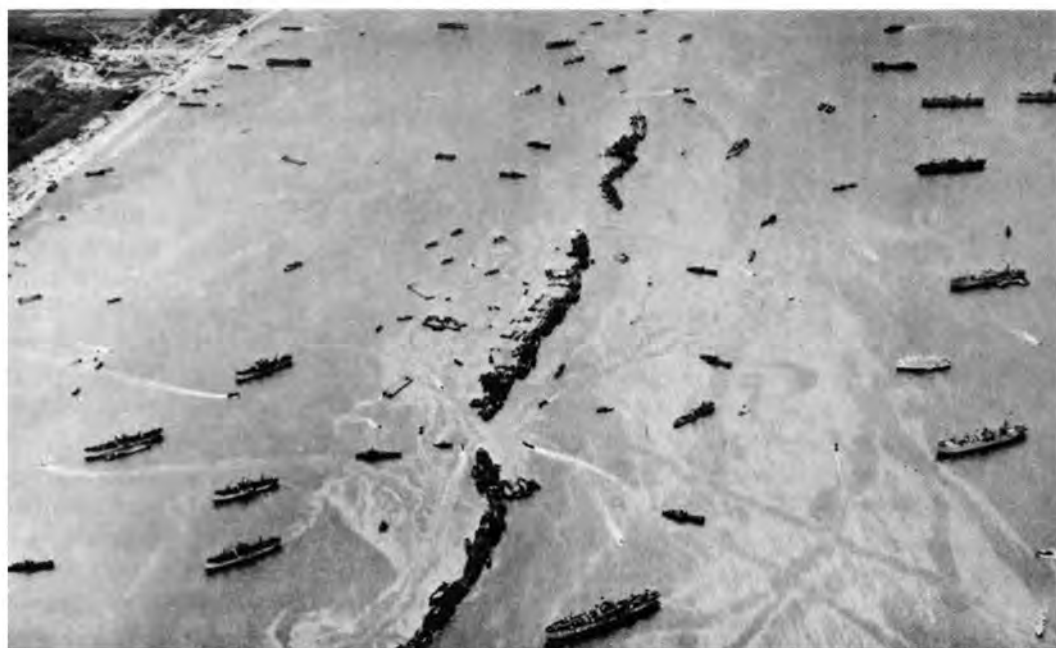
ARTIFICIAL PORT AT OMAHA BEACH. Unloading equipment (above) on pier off Vierville Draw. Pier on right is under construction. Both were destroyed during the storm on 21 June. Breakwater of sunken ships (below). At upper left is les Moulins draw.
