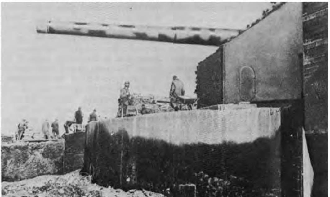
ENEMY COAST ARTILLERY in the Pas-de-Calais area. Heavy concrete casemate under construction ( above ), and ( below ) laborers at work on casemate.
