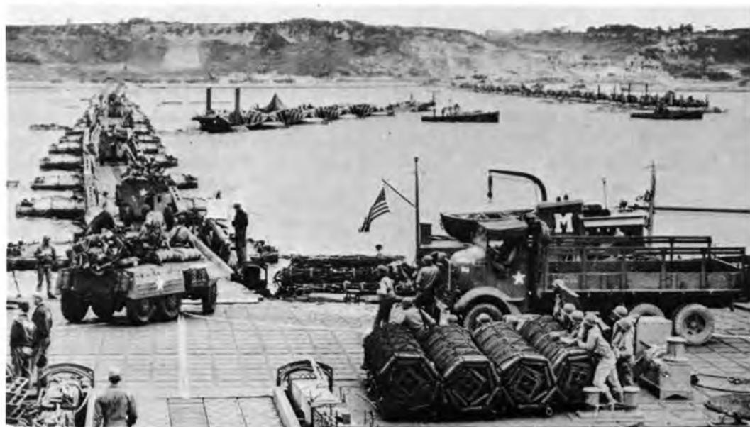
ARTIFICIAL PORT AT OMAHA BEACH. Unloading equipment (above) on pier off Vierville Draw. Pier on right is under construction. Both were destroyed during the storm on 21 June. Breakwater of sunken ships (below). At upper left is les Moulins draw.
