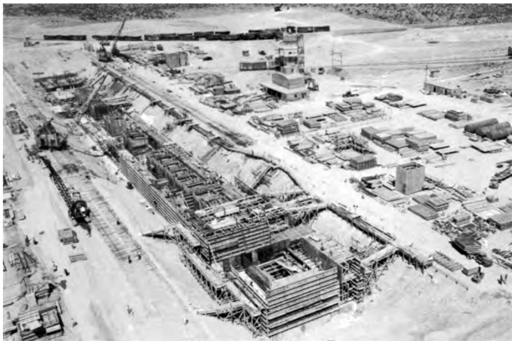
CHEMICAL SEPARATION PLANT UNDER CONSTRUCTION AT HEW
