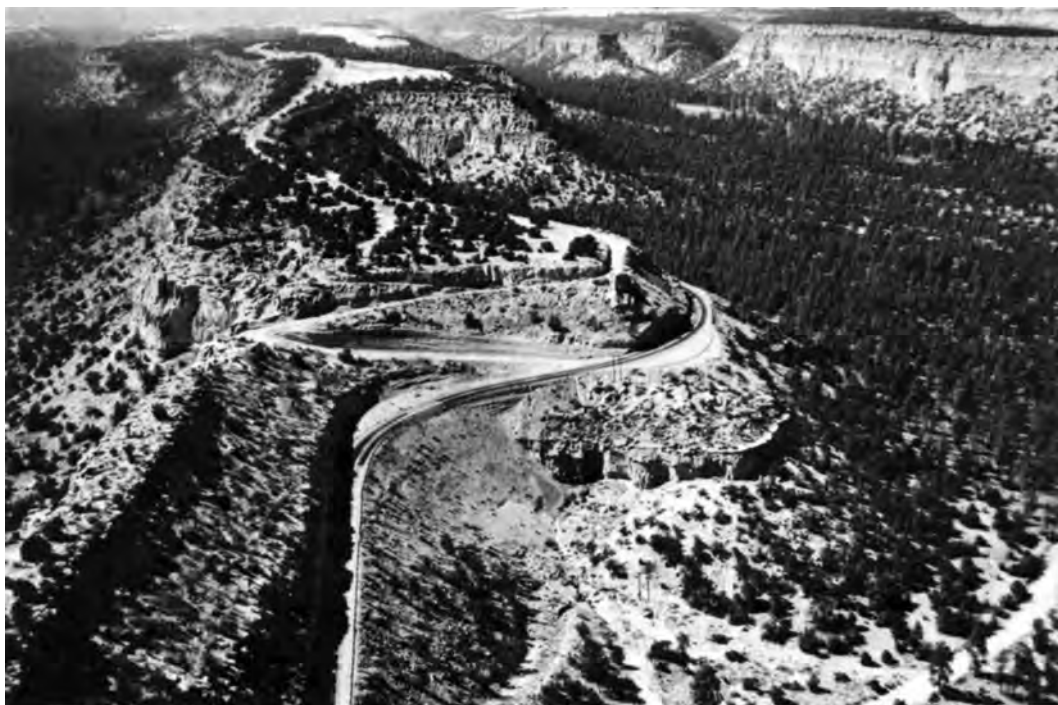
IMPROVED SANTA FE-LOS ALAMOS ROAD, ascending to the Pajarito Plateau from the Rio Grande valley
