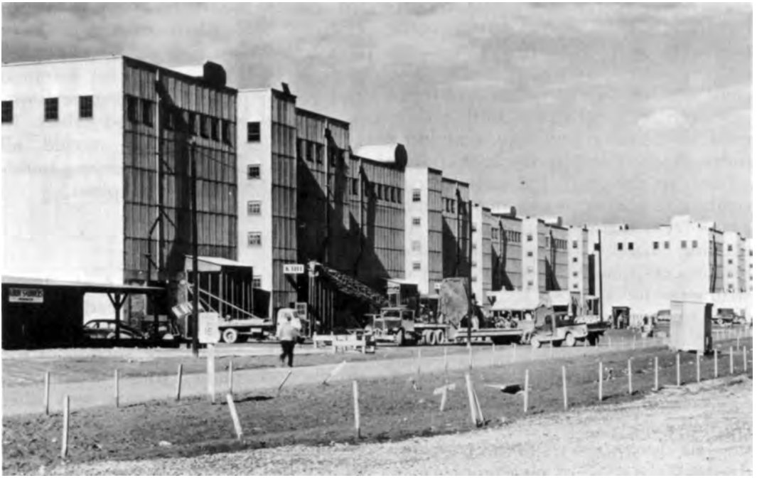
COMPLETED PLANT SECTION with corrugated steel sheathing
