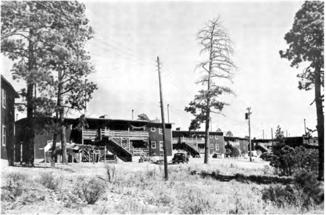
FOUR-FAMILY APARTMENT UNITS AT LOS ALAMOS
