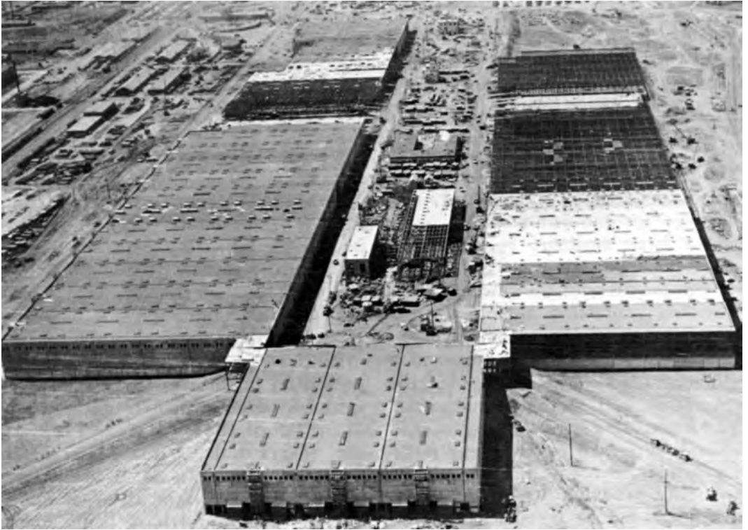
GASEOUS DIFFUSION PLANT UNDER CONSTRUCTION AT CEW
