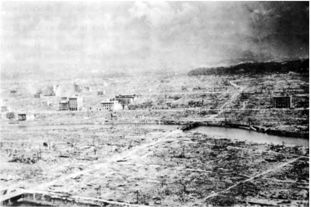
PHYSICAL DAMAGE AT HIROSHIMA
