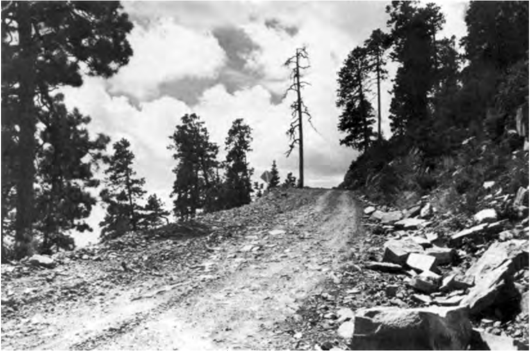
UNIMPROVED SANTA FE-LOS ALAMOS ROAD
