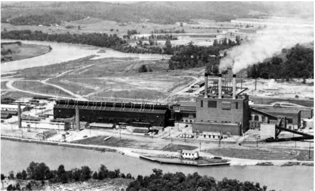
LIQUID THERMAL DIFFUSION PLANT ( long, dark building ) AT CEW. The adjacent K-25 power plant drew water from the Clinch River.
