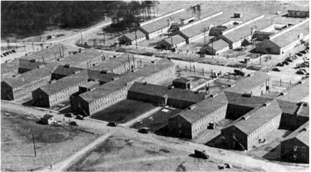
CEW TRAINING FACILITIES ( background ), where electromagnetic plant employees received preliminary instruction. District headquarters buildings are in the foreground.
