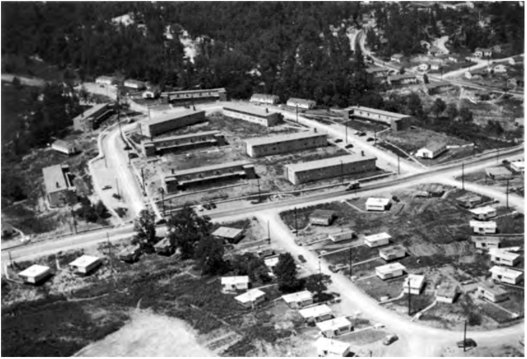
PREFABRICATED HOUSES ( foreground ) AND APARTMENT DWELLINGS ( center ) AT CEW
