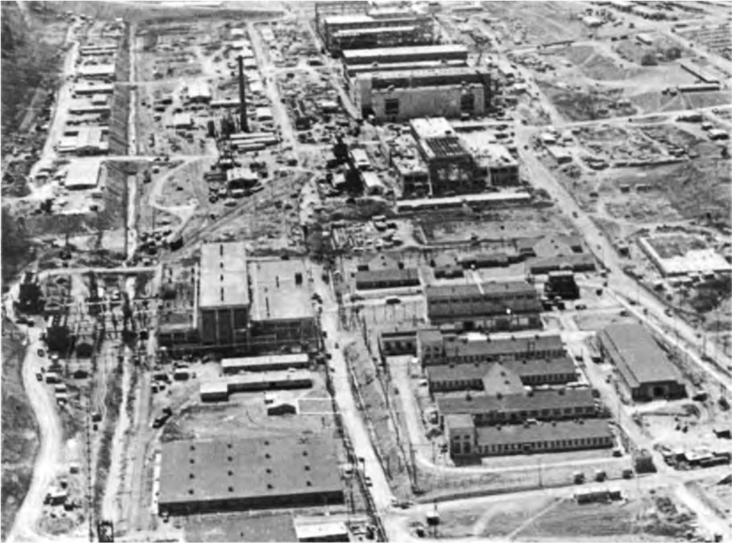
ELECTROMAGNETIC PLANT UNDER CONSTRUCTION
