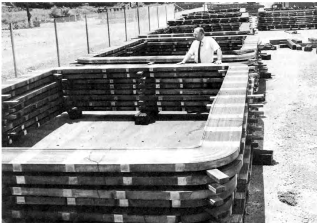
SILVER-WOUND MAGNET COILS FOR THE ELECTROMAGNETIC PROCESS
