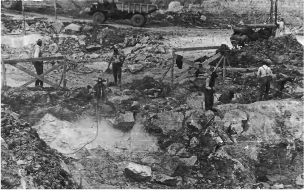
EXCAVATION OF TYPICAL ROCKY SUBSTRATUM AT THE TENNESSEE SITE
