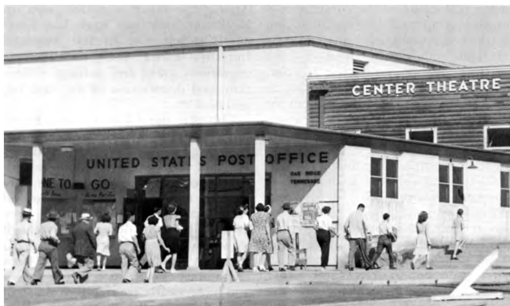
MAIN POST OFFICE AND THEATER IN OAK RIDGE
