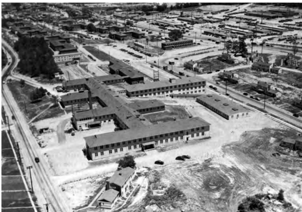
OAK RIDGE HOSPITAL ( multiwinged structure in foreground )
