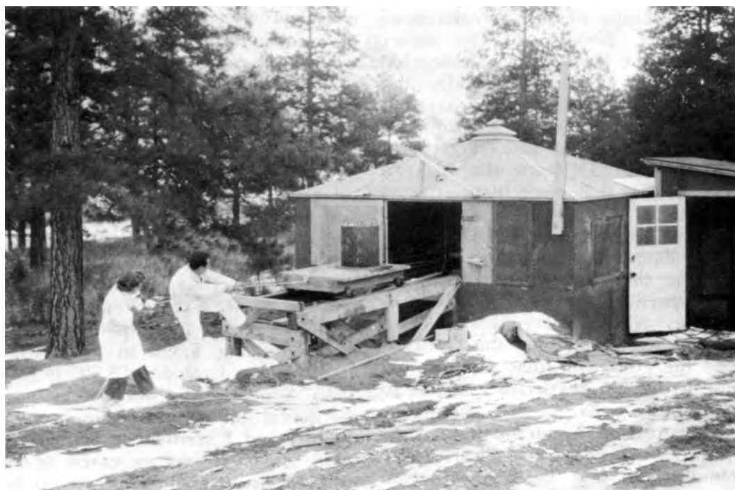
HAZARDOUS MATERIALS STORAGE AREA AT LOS ALAMOS. Technicians are removing lead-lined container.
