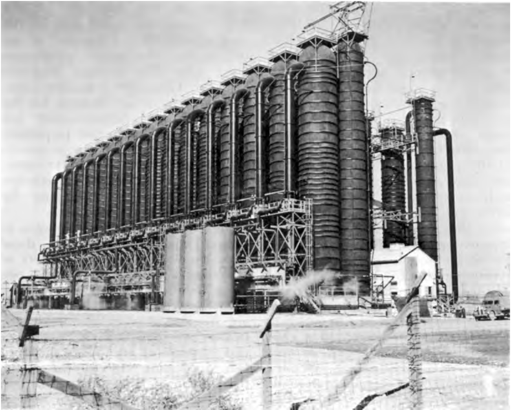
HEAVY WATER PRODUCTION PLANT AT THE WABASH RIVER ORDNANCE WORKS
