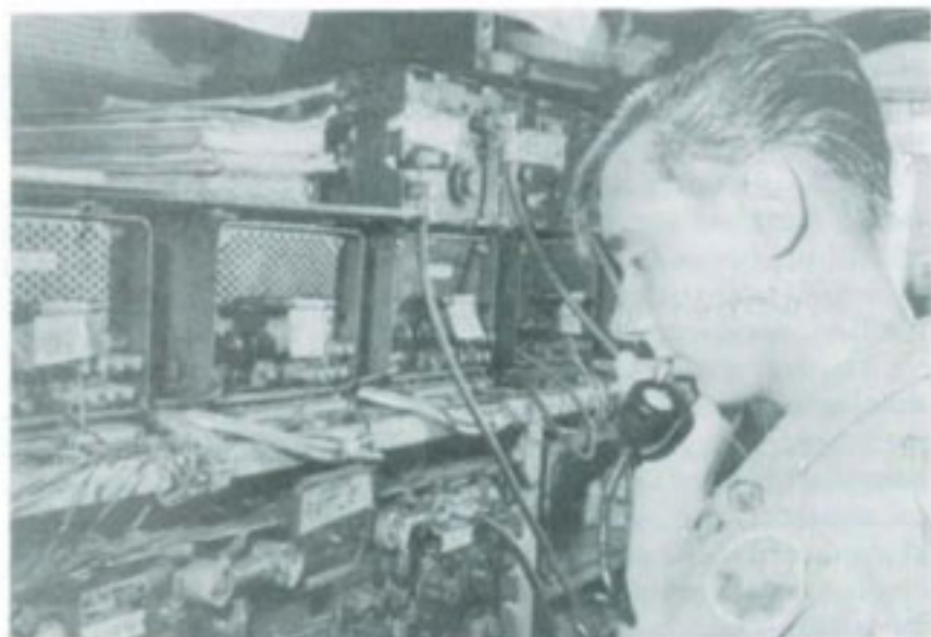
AN/GRC/TCC-3 MULTICHANNEL EQUIPMENT aboard the Benewah.
