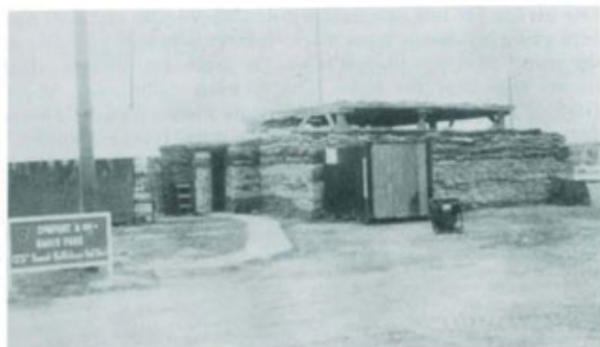
HIGH FREQUENCY RADIO BUNKER at 25th Infantry Division headquarters in Cu Chi. Antenna mast was made from artillery power canisters.
