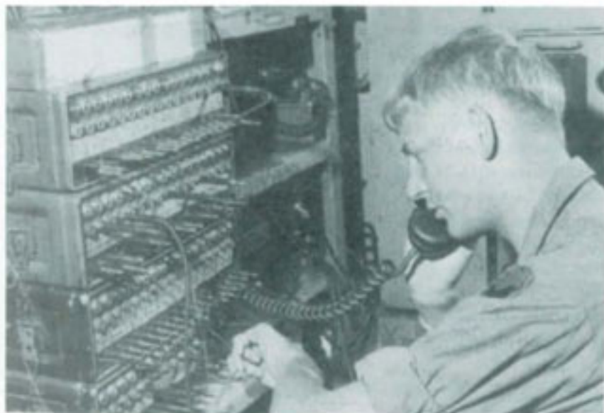
SB-22 SWITCHBOARD aboard the Benewah.
