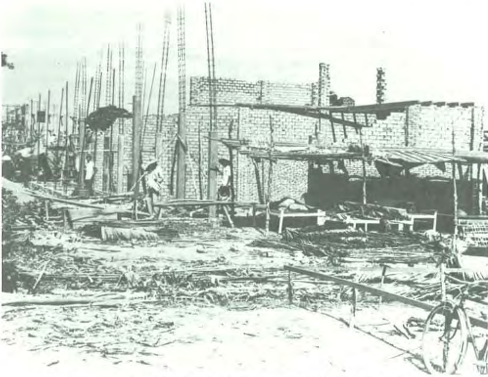
Agroville Under Construction at Vi Thanh, Phong Dinh Province.
