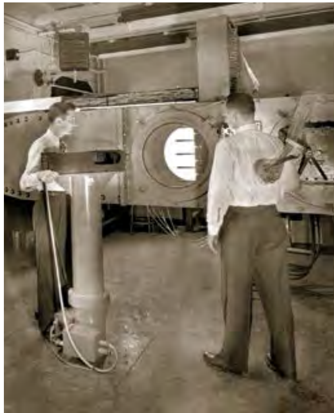
Image 113: A technician operates a Schlieren camera to view the airflow dynamics inside the 24- by 24-inch test section of one of the Stack Tunnels (GRC-1949-C-24977).
