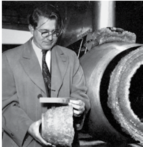
Image 103: Abe Silverstein measures ice buildup on the Westinghouse J34 engine (GRC-1948-C-20836).
