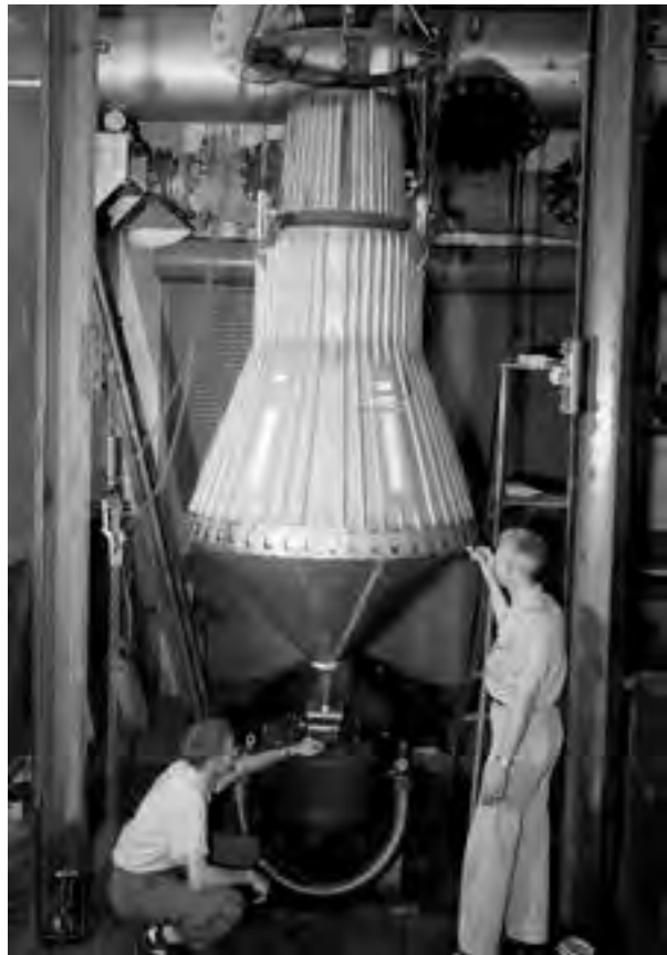
Image 175: Technicians in the Fabrication Shop align the Mercury capsule afterbody with its pressure chamber in May 1959 (GRC-1959-C-50759).
