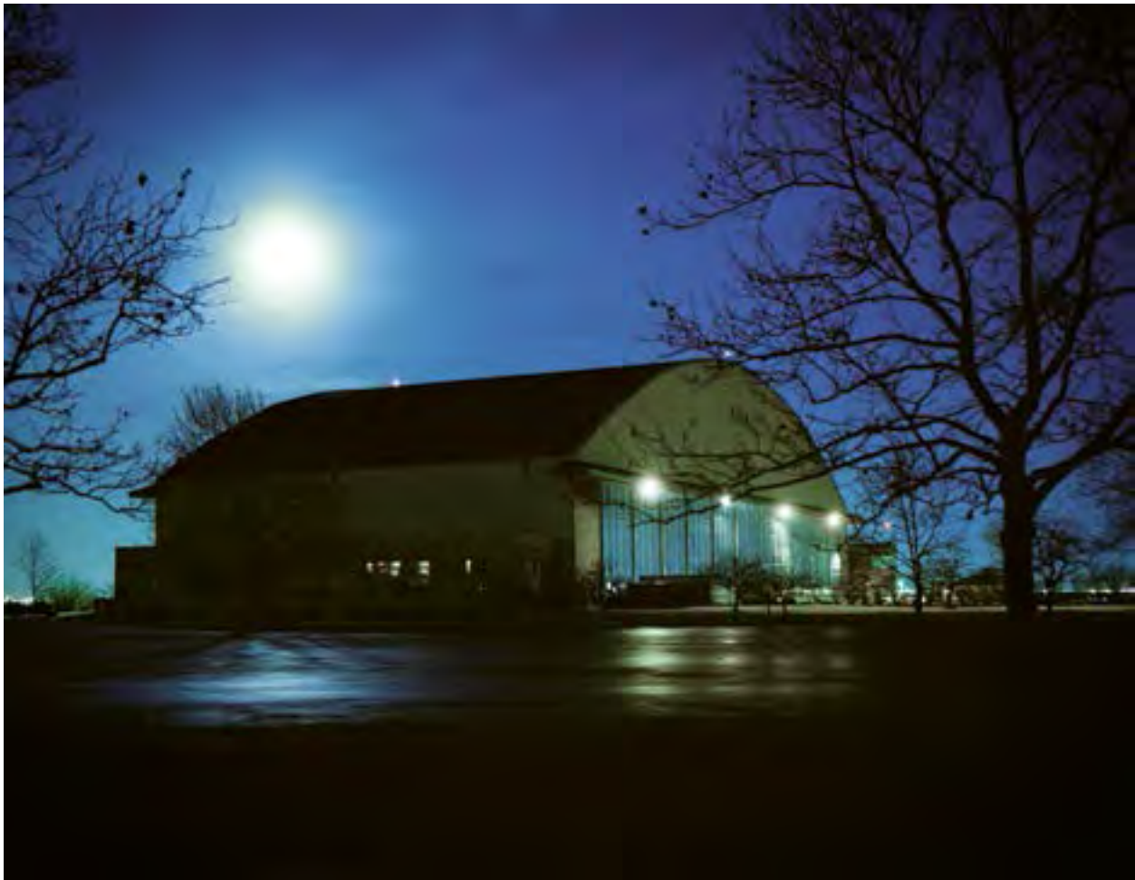
Image 289: The Lewis hangar in November 1981 (GRC-1981-C-05731).
