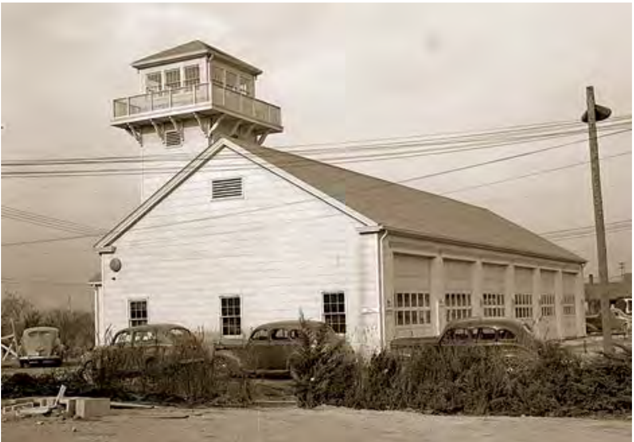
Image 54: PBOW fire station located near Taylor and Columbus avenues, c1941 (GRC-2015-C-06564).
