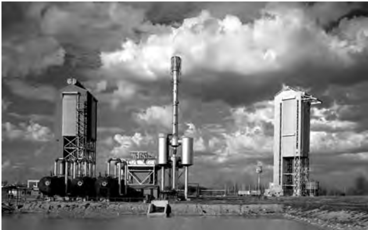
Image 198: The B-1 and B-3 test stands, 135 and 210 feet tall, could test different components of high-energy rocket engines under flight conditions (GRC-1964-C-01310).
