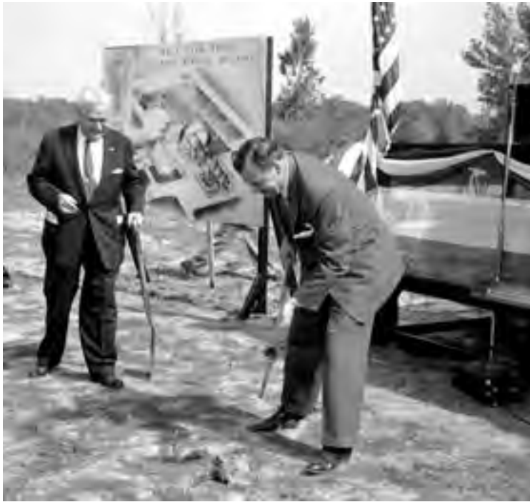
Image 134: Ray Sharp and Congressman Albert Baumhart break ground for the Plum Brook Reactor Facility in September 1956. The pick and shovel were the same as those used for the AERL groundbreaking in January 1941 (GRC-1956-C-43033).
