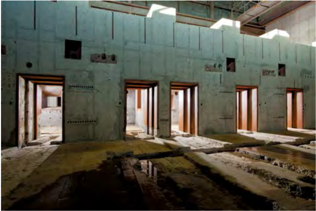
Image 355: The gutted remains of the reactor's Hot Lab, which was used to remotely examine irradiated test specimens (NASA SPF 1697).
