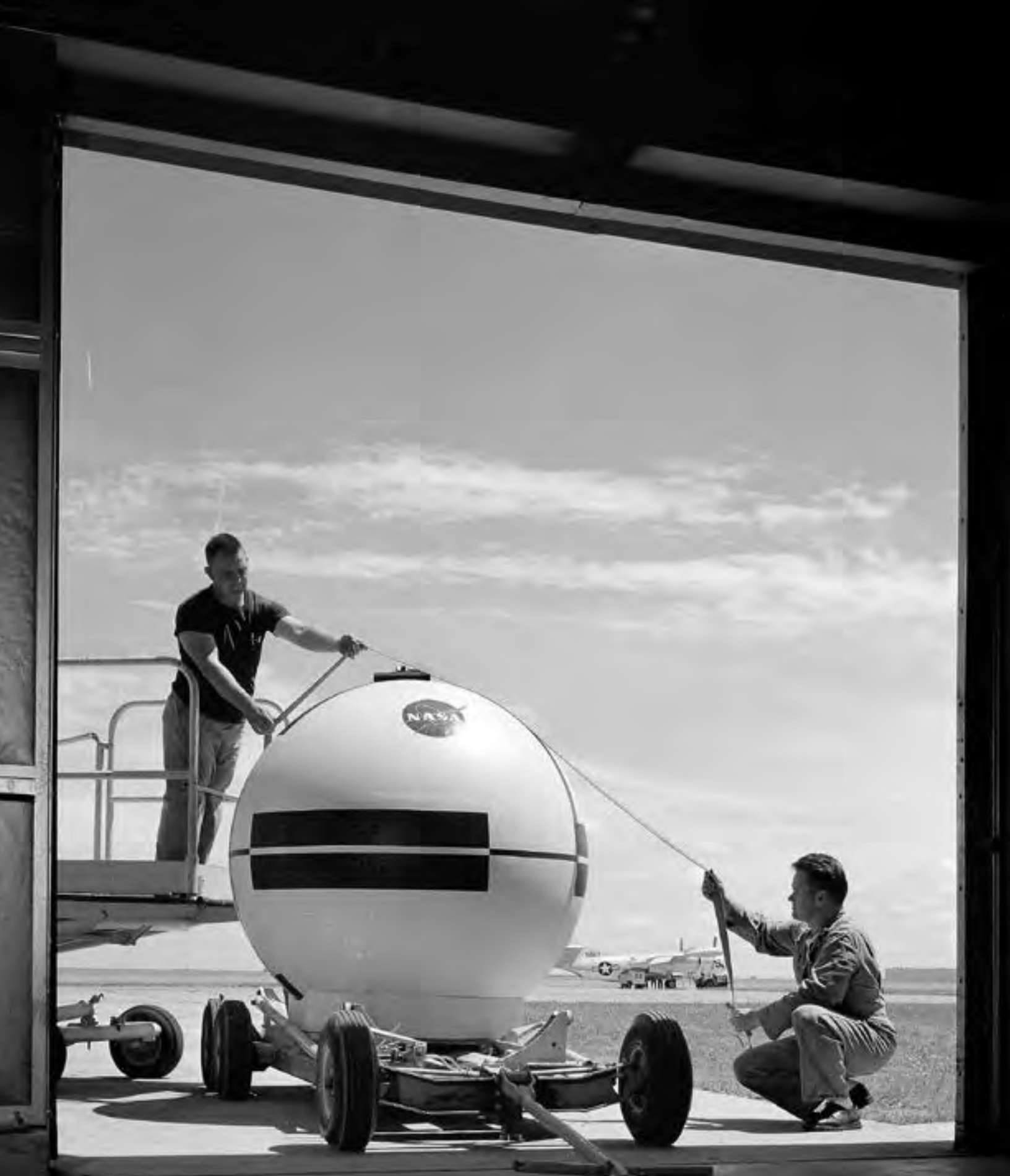
Image 411: Technicians prepare a spherical liquid-hydrogen tank in June 1960 to study the fluid's behavior in low gravity during a flight on the center's AJ-2 Savage aircraft (GRC-1960-C-53861).
