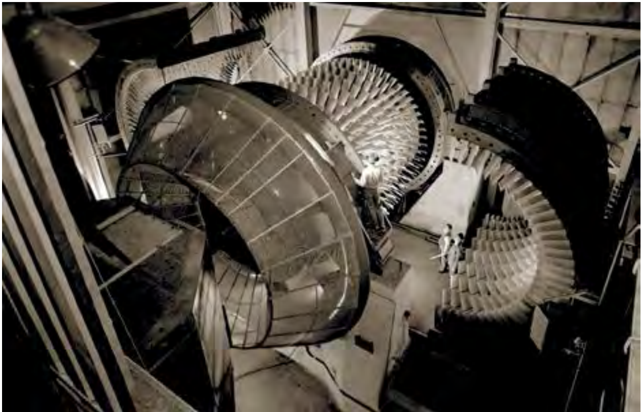
Image 117: The seven-stage axial compressor that powers the 8×6. The compressor was driven by three electric motors with a total output of 87,000 horsepower, resulting in airspeeds from Mach 0.36 to 2.0 (GRC-1949-C-23277).
