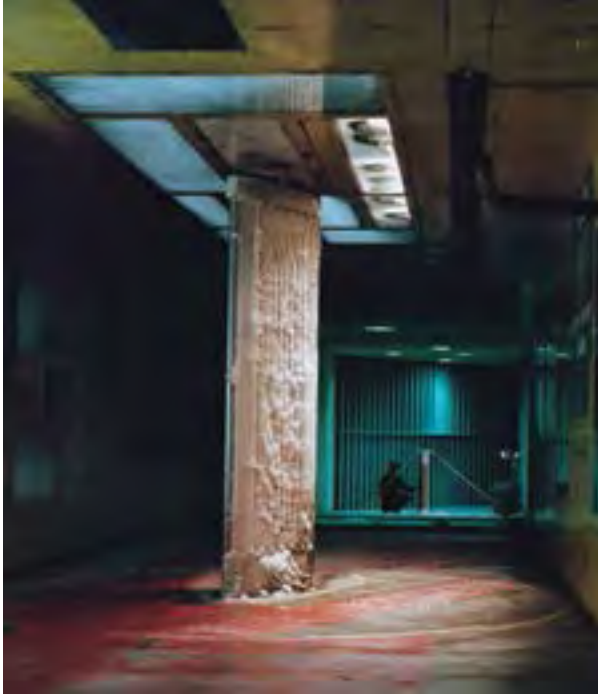
Image 298: A prototype turning vane for the new AWT installed in the IRT during December 1985 (GRC-1985-C-09342).
