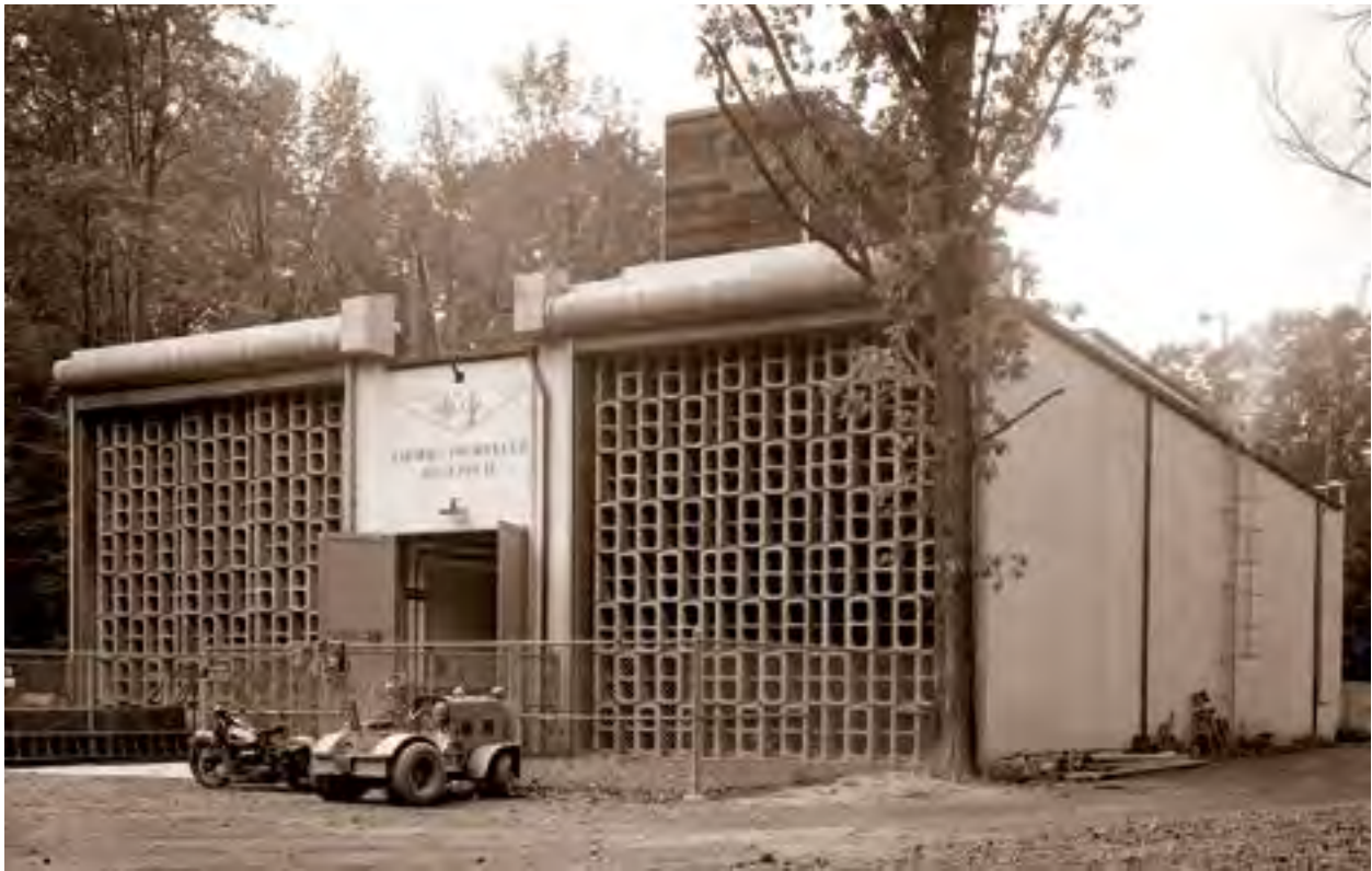
Image 34. In May 1942 the Prop House became the first operating facility at the AERL. It contained four test cells designed to study large reciprocating engines. Researchers tested the performance of fuels, turbochargers, water-injection, and cooling systems here during World War II. The facility was also used to investigate a captured German V-1 buzz bomb during the war (GRC-1942-C-01134).
