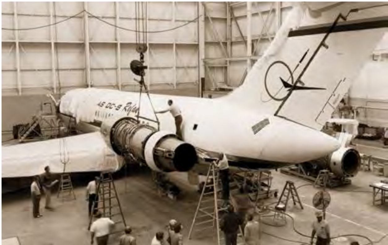
Image 272: A Refan engine installed on a DC-9 for a ground test in January 1975 (GRC-1975-C-00104).
