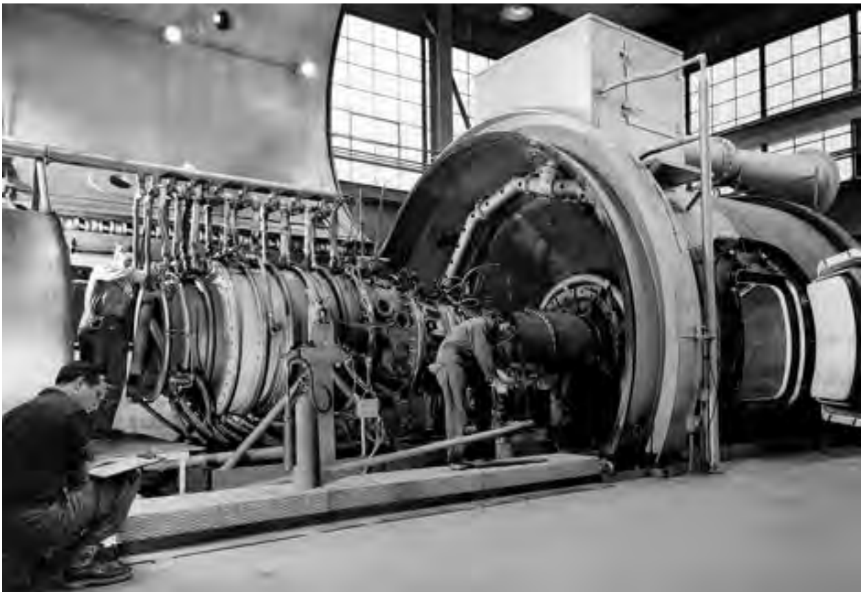
Image 145: A Wright Aeronautical XRJ-47-W-5 ramjet installed in a PSL test chamber for the Navaho program (GRC-1952-C-30961).
