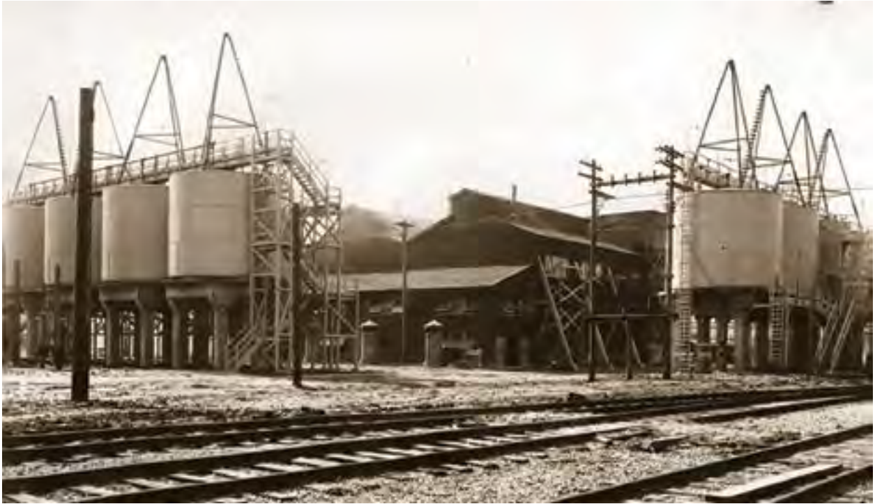
Image 53: One of three acid-producing facilities at the PBOW. The acid was used to manufacture TNT and DNT, c1941 (GRC-2015-C-06540).
