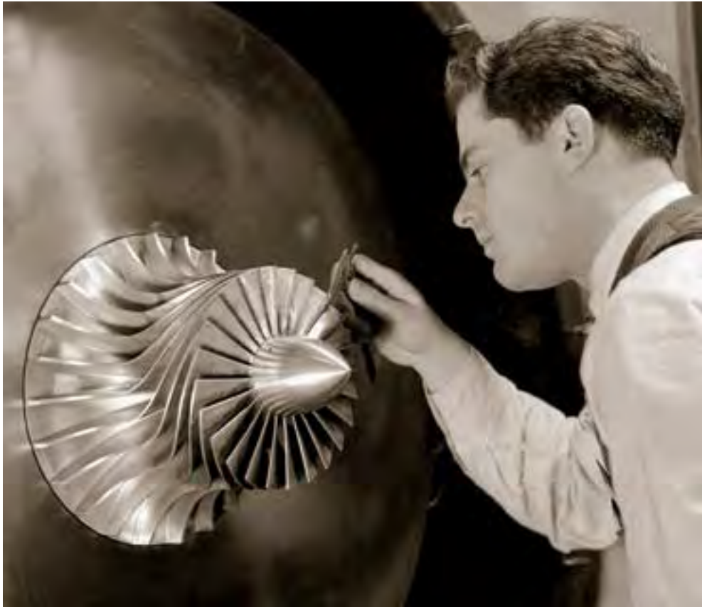
Image 78: An AERL metallurgist examines a supercharger in January 1944 (GRC-1944-C-03814).
