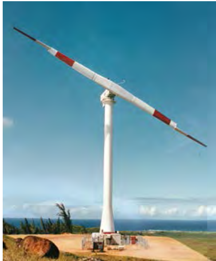
Image 264: The Boeing 7.2-MW wind turbine began operation in Oahu in July 1987 (GRC-1987-C-05991).
