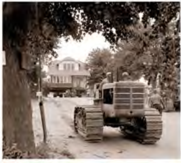
Image 27: Crews remove a farmhouse from the PBO site in summer 1941 (GRC-2015-C-06561).
