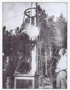
The GIRD team is shown here in 1933 feeding liquid oxygen to the "09." the first Soviet liquid-propellant rocket. From left to right are Sergey Korolev, Nikolay Yefremov, and Yuriy Pobedonostsev.
