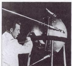
The PS-1 satellite is shown here on a rigging truck in the assembly shop in the fall of 1957 as a technician puts finishing touches on it.
