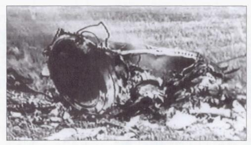
This shows the wreckage of the Soyuz I descent apparatus immediately after the crash. Cosmonaut Vladimir Komarov's body was still buried within the wreckage at the time of this photograph. (Rudy, Inc., via Quest magazine)
