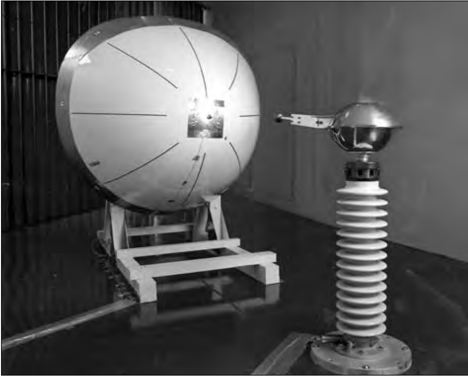
Figure 8–2. Lightning generator and radome in IRT, 1955. (NASA C-1995-4467)
