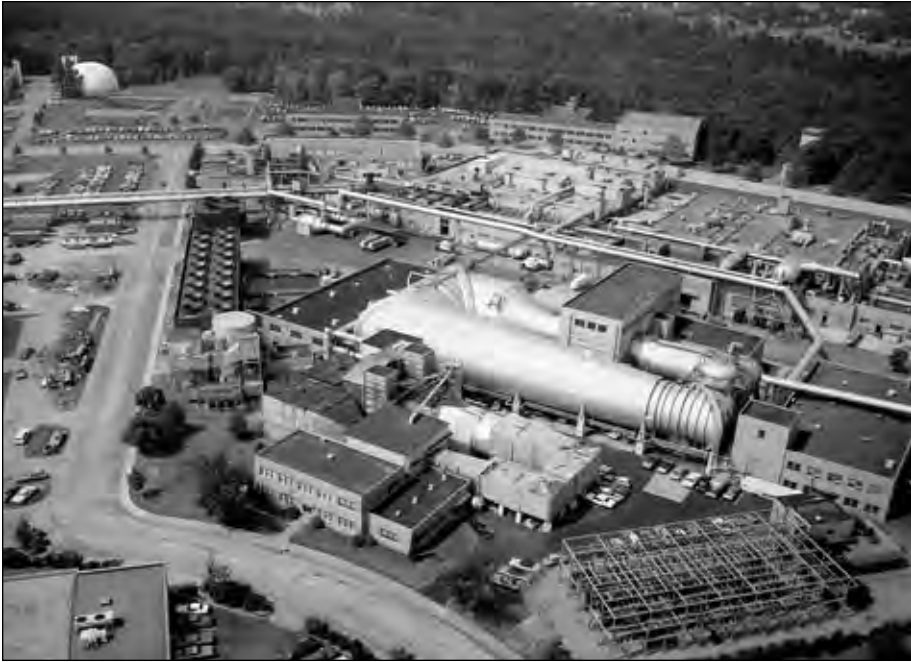
Figure 5-1. Overhead view of the IRT and AWT, 1971. (NASA C-71-3281)
