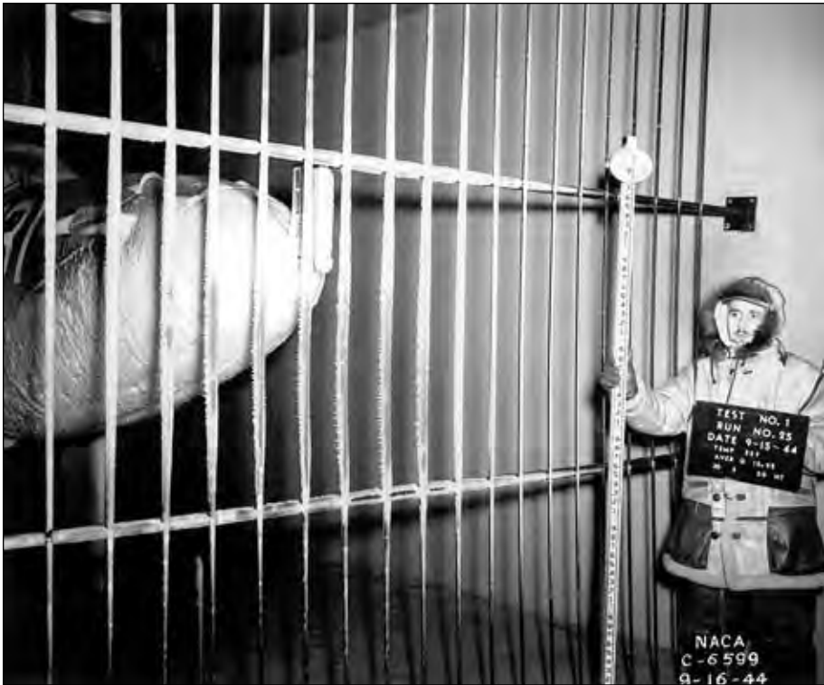
Figure 3-2. Propellor with internal heaters after icing run, 15 September 1944. (NACA C-6599)
