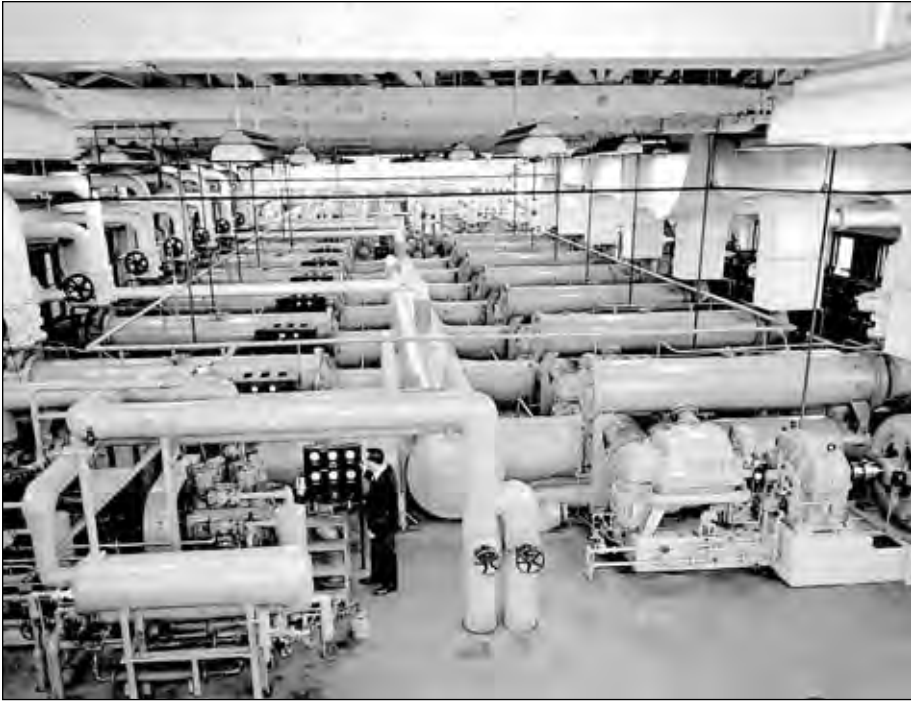
Figure 4–9. Refrigeration plant for the IRT and AWT, 1 March 1951. (NACA C-27262)
