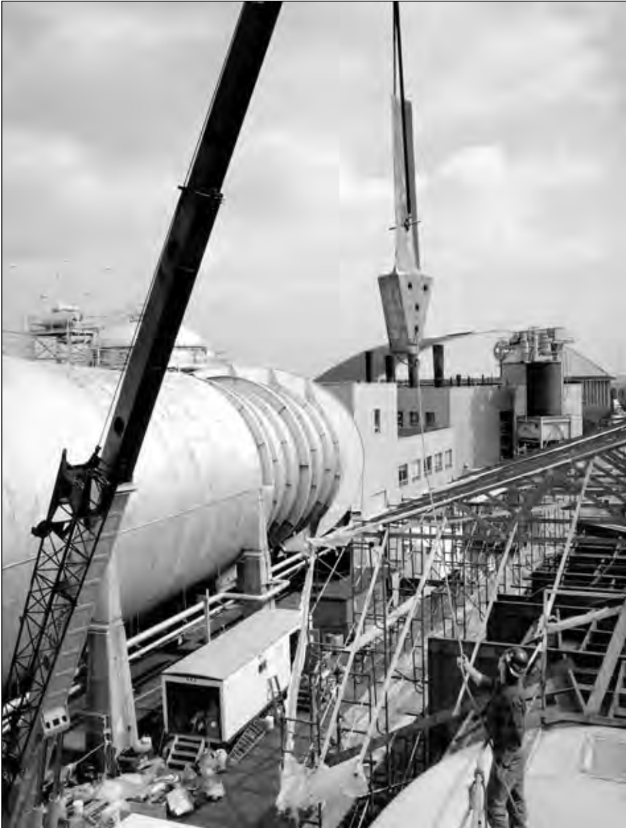
Figure 7-3. IRT renovation, 1993. (NASA C-93-7170)
