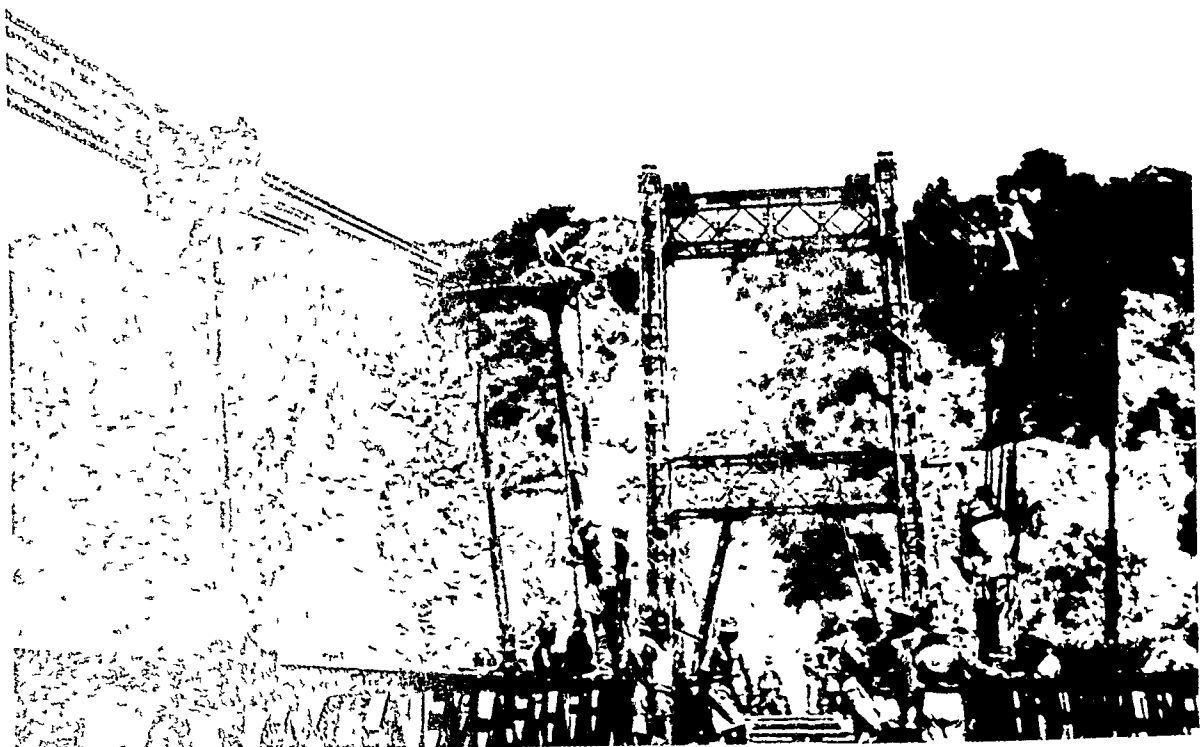
Bridge under construction by Indian Engineers at Beri Pattan
