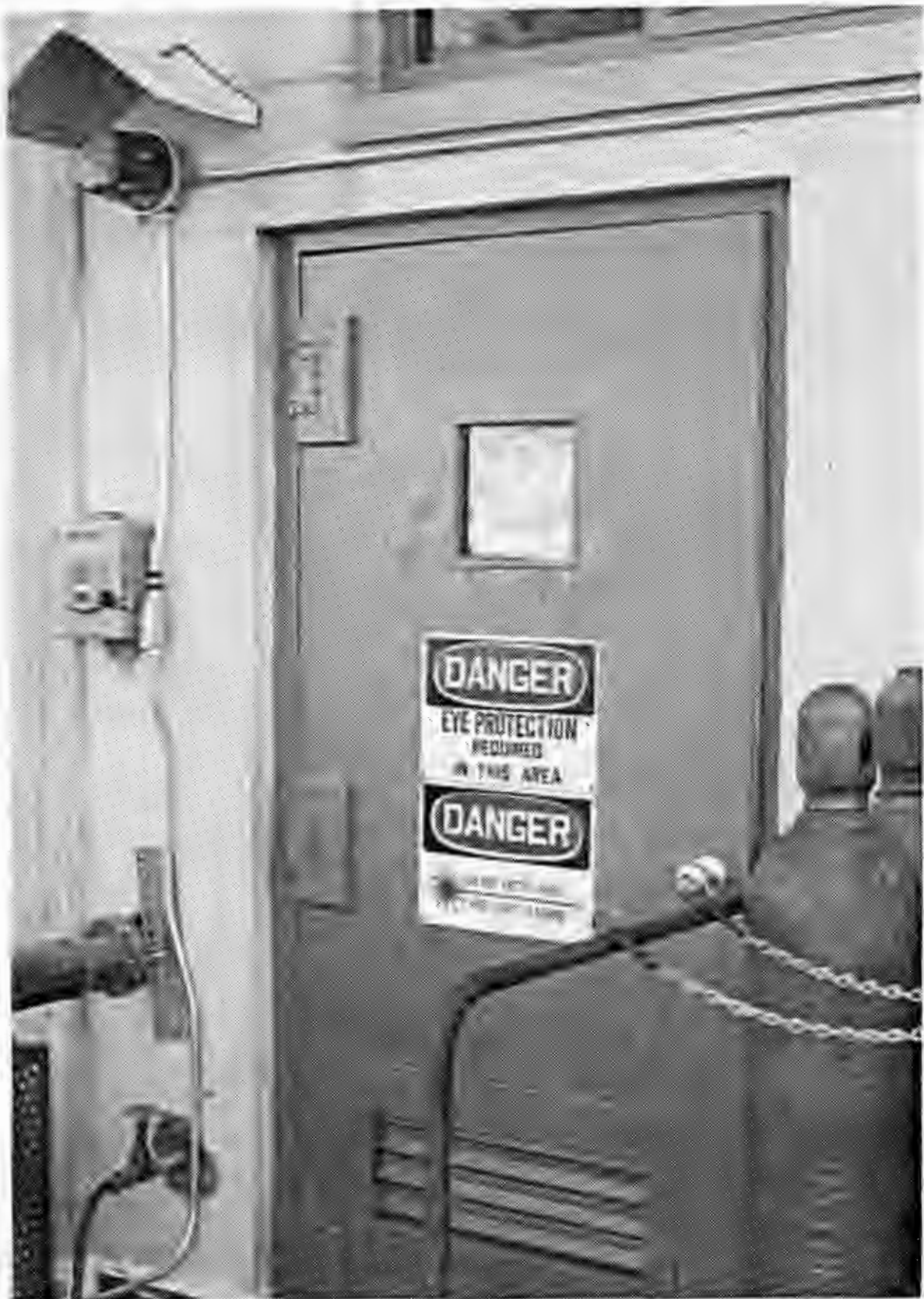
Figure 10 - LASER ROOM-EXTERNAL VIEW
