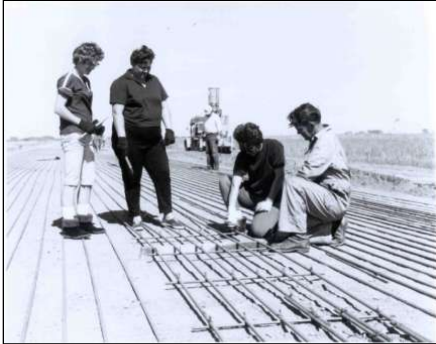
Figure 72 - Continuously reinforced concrete (CRC) steel placement on chairs
