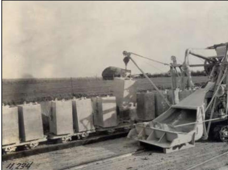
Figure 20 - Lifting rail box into skip hoist – Wapello County 1926
