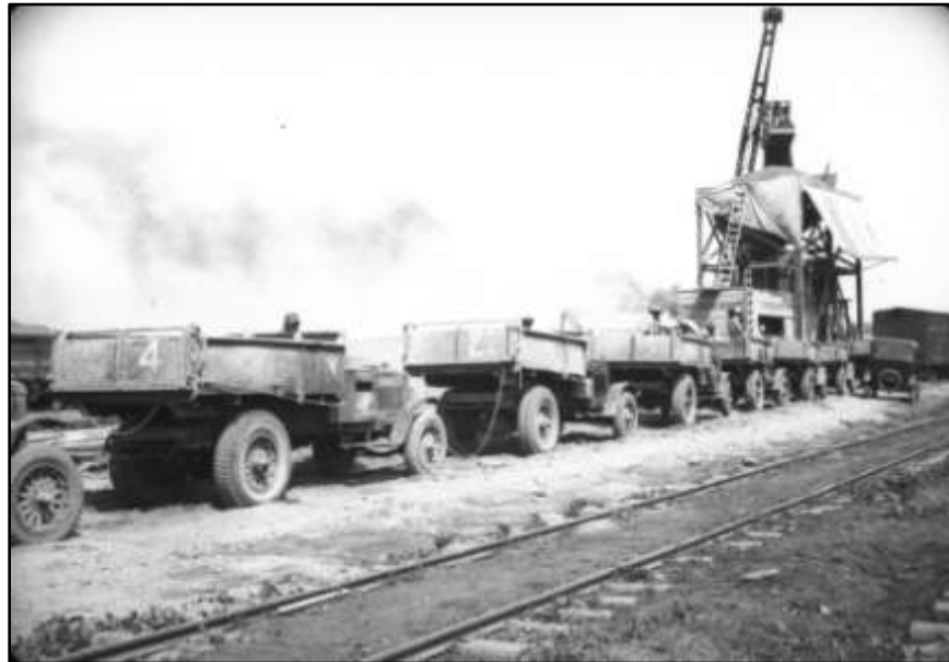
Figure 16 - Trucks lined up at aggregate batch plant - Woodbury County 1921
