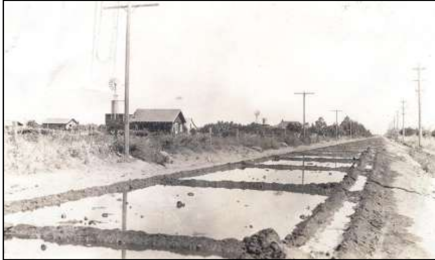
Figure 46 - Curing by ponding - Mitchell County 1930s
