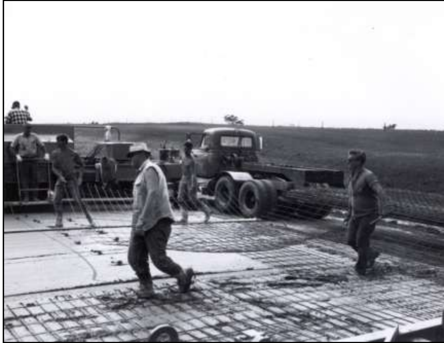
Figure 71 - Mesh reinforcement - Dallas County I-80 1966
