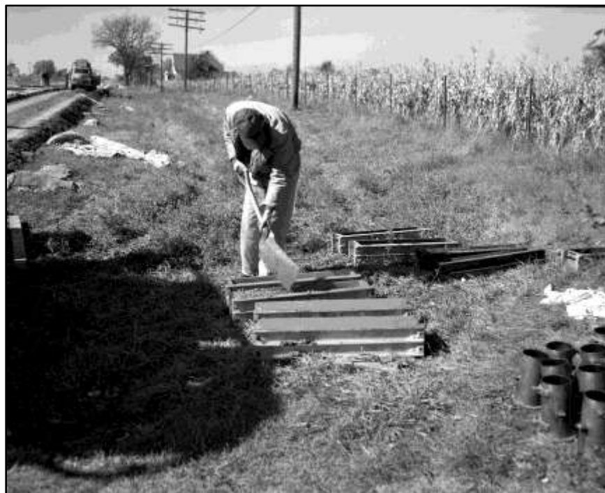
Figure 50 – Worker casting flexural strength specimens
