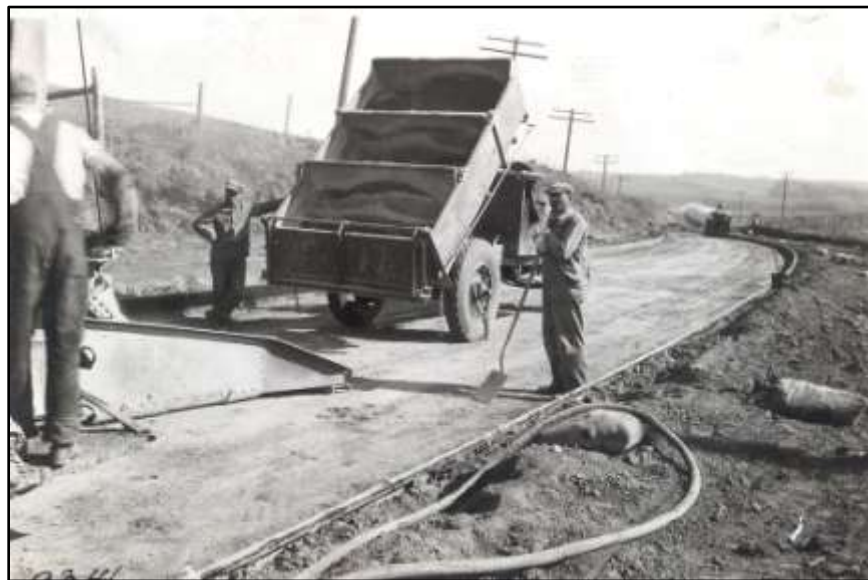
Figure 17 - Truck dumping into skip hoist - Woodbury 1921
