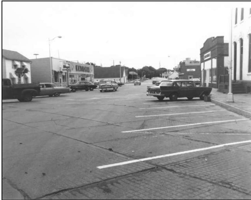
Figure 1 Le Mars city street built 1904 - picture 1950s
