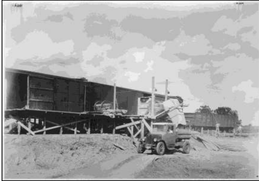
Figure 18 - Bulk cement dumping into truck – Howard County 1931
