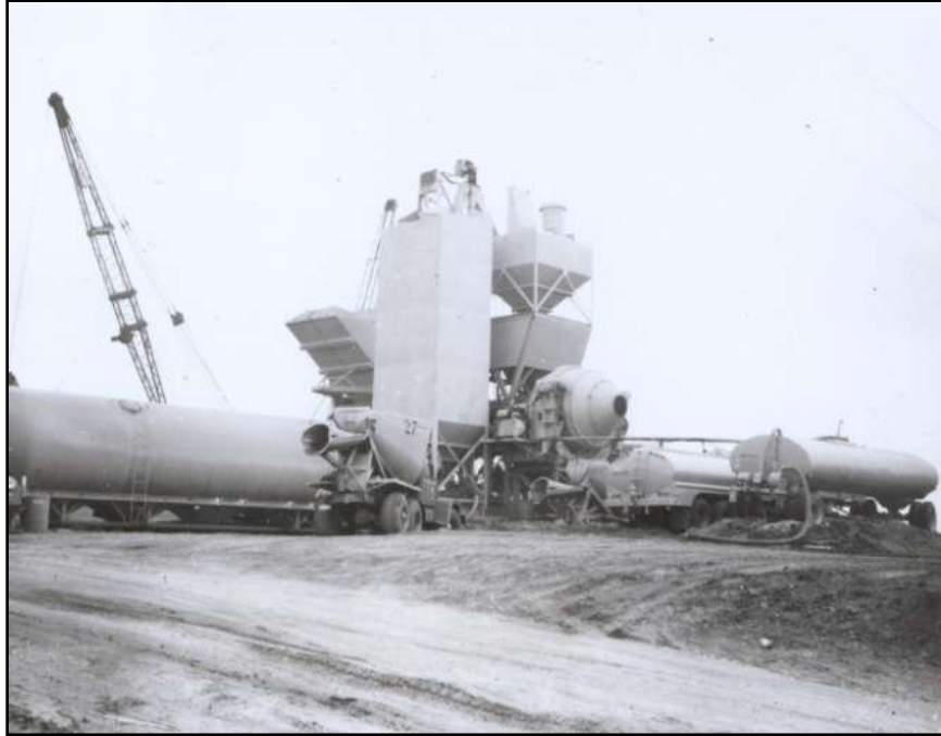
Figure 23 - Central batch plant – Cass County I-80 1965
