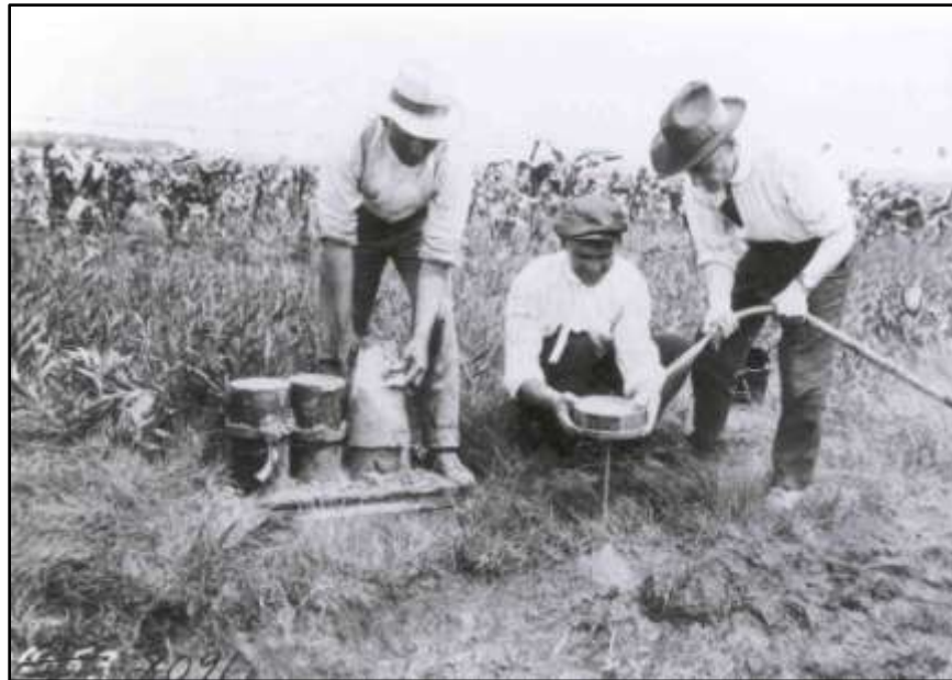
Figure 12 - Testing slump and cylinders – Dallas County 1921
