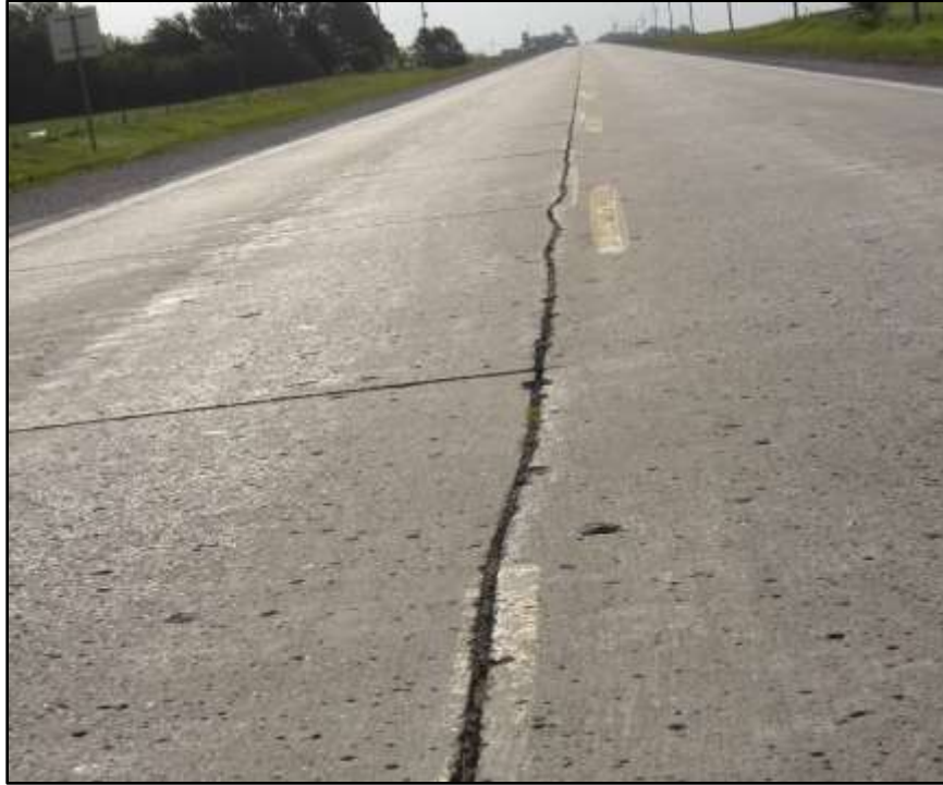
Figure 58 – Longitudinal joint with continuous placed parting strip – U.S. 30 Greene County
