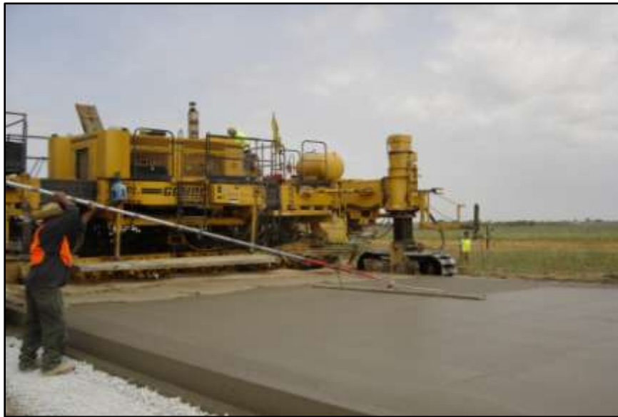
Figure 34 – Gomaco slip form paver - Henry County 2005
