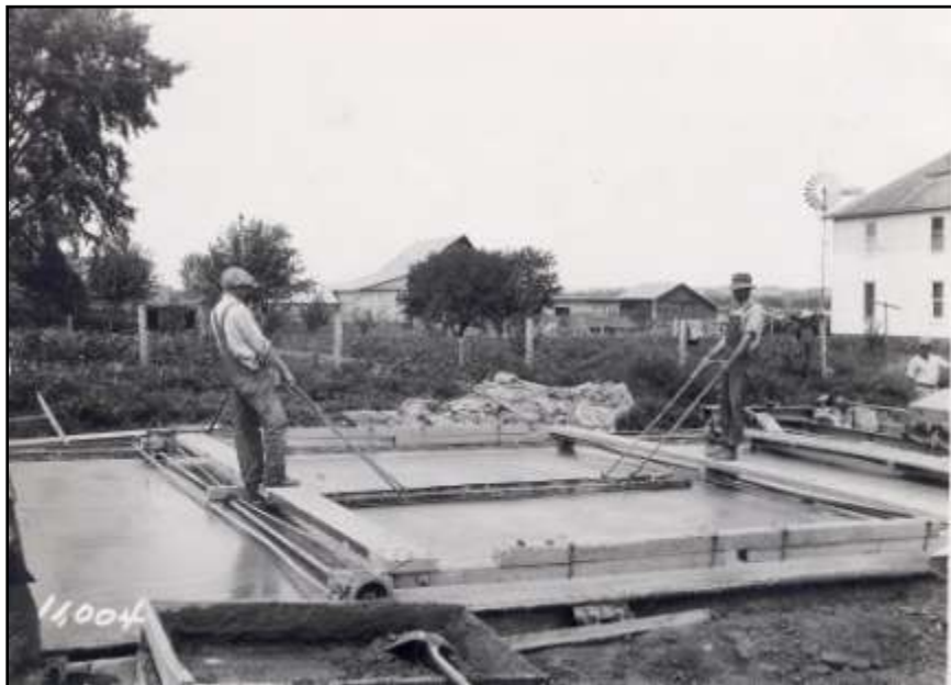
Figure 40 - Longitudinal finishing – Polk County 1926
