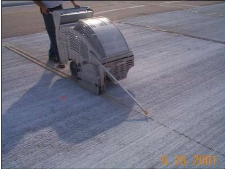
Figure 60 - Early entry sawing transverse joint
