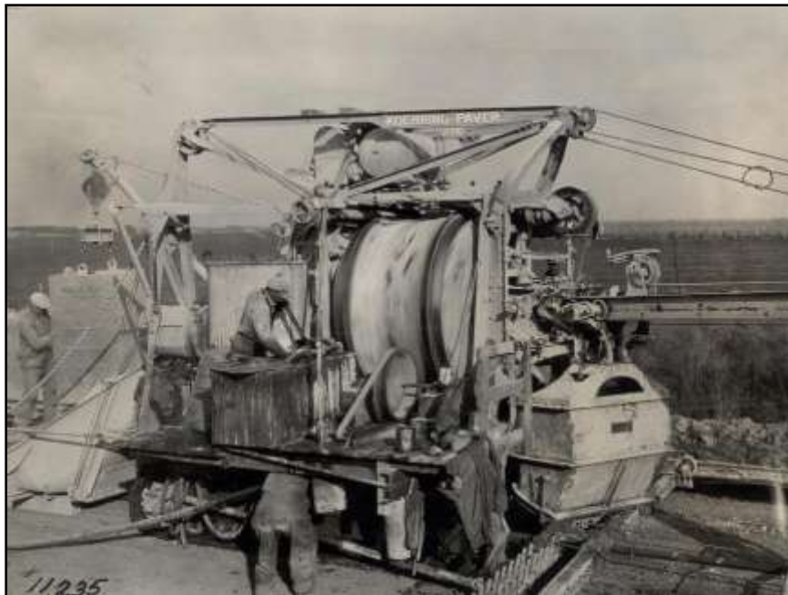
Figure 21 - Koehring paver mixer – Wapello County 1926
