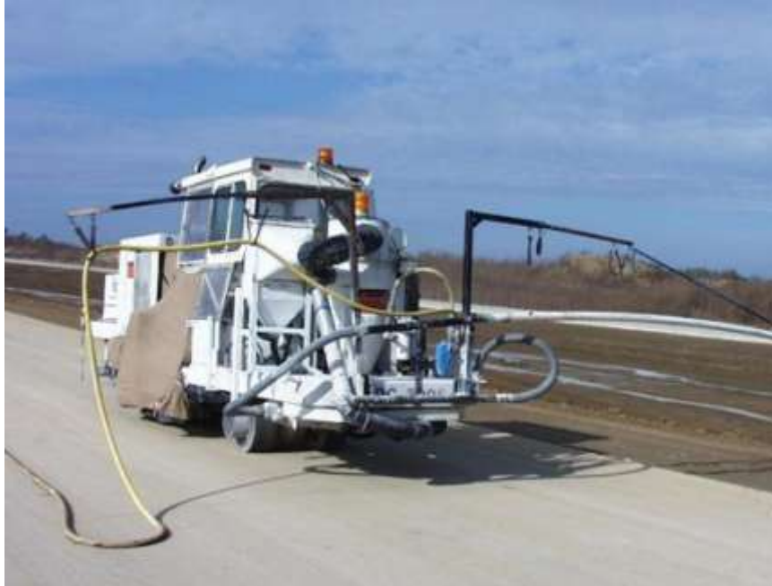
Figure 64 – Surface correction with diamond grinding equipment
