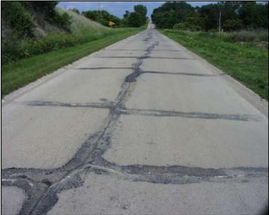
Figure 52 - Old U.S. 20 Woodbury County 1921 - no jointing
