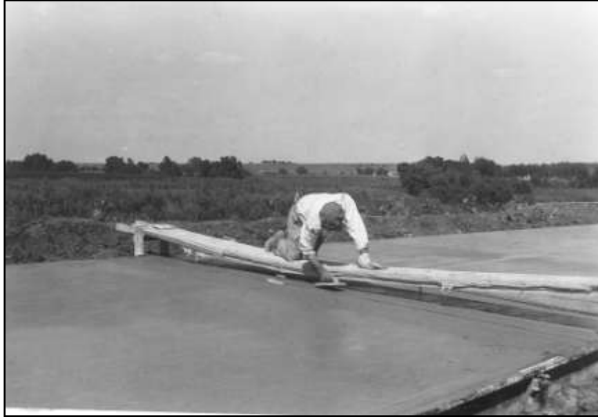
Figure 55 - Finishing expansion joint – Montgomery County 1930
