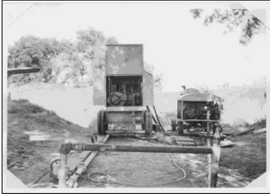
Figure 14 - Water lines and pumping equipment – Shelby County 1930s
