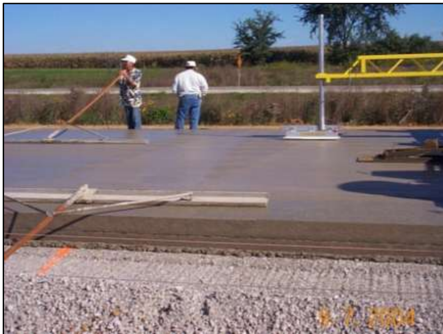
Figure 79 – Noncontact smoothness profile equipment (Ames Engineering)
