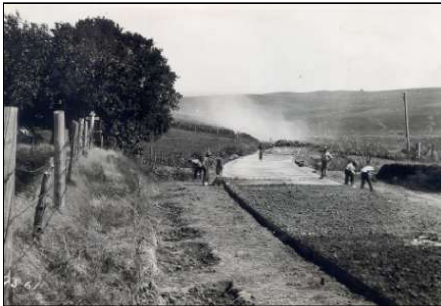
Figure 45 - Earth curing - Woodbury County 1921
