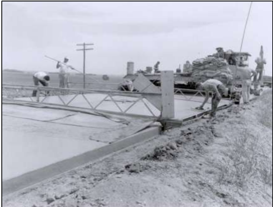
Figure 31 - Quad City slip form paver – Palo Alto County 1957
