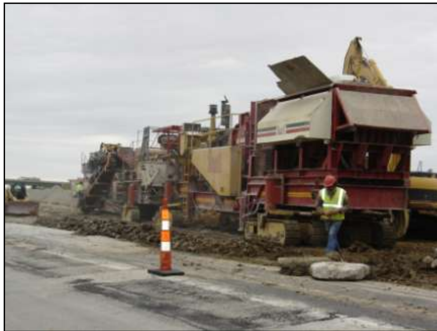
Figure 7 - "Paradigm" Mobile Crushing Equipment
