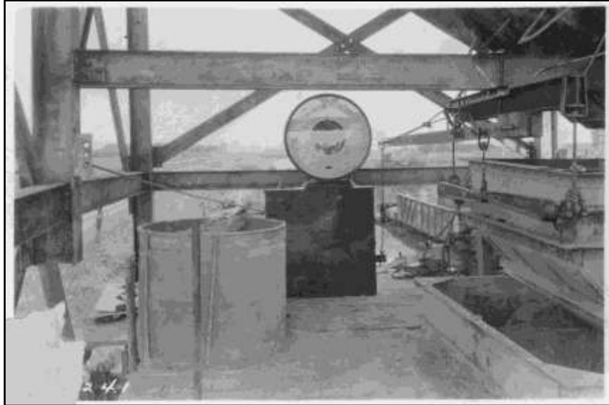
Figure 11 - Weigh scale and aggregate hopper – Woodbury County 1921
