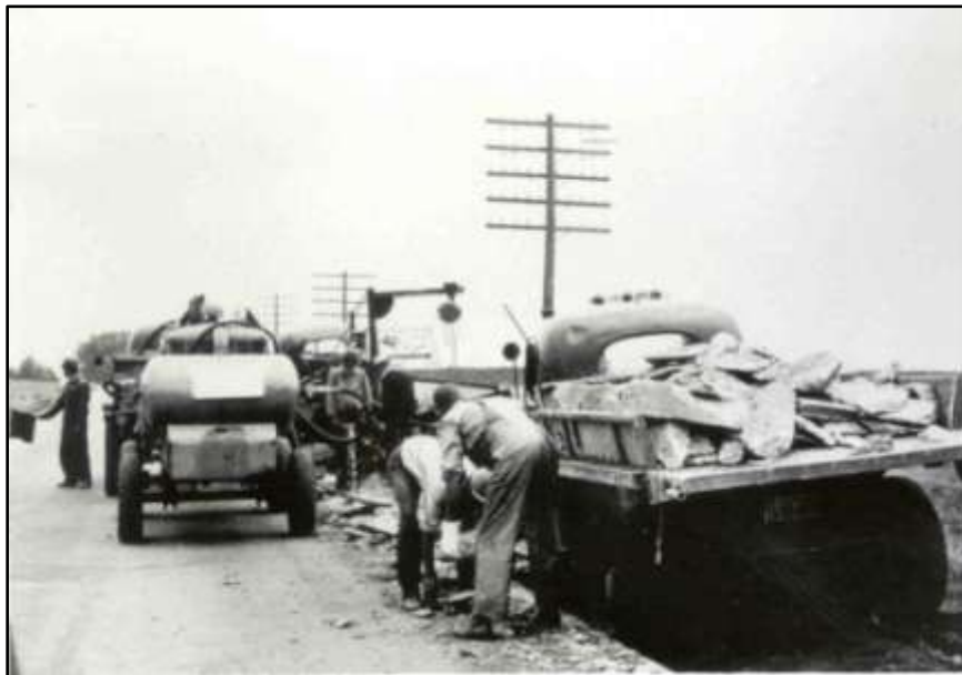
Figure 70 - Curb removal and widening – U.S. 69 Polk and Story counties 1948
