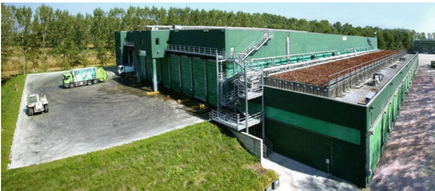
Fig. 2 View of a bio-drying system located in Italy, similar to the one described
