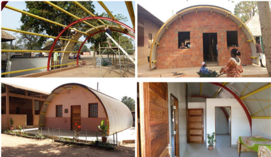
Fig. 8 Borboleta construction phases: structures, non-load-bearing wall, finishing, and interiors
