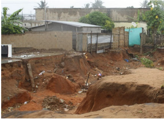
Fig. 3 Example of the harmful effects of uncontrolled urbanisation. Episodes of soil erosion due to torrential rains in a typical shanty town in the village of Maxixe (author's photos)
