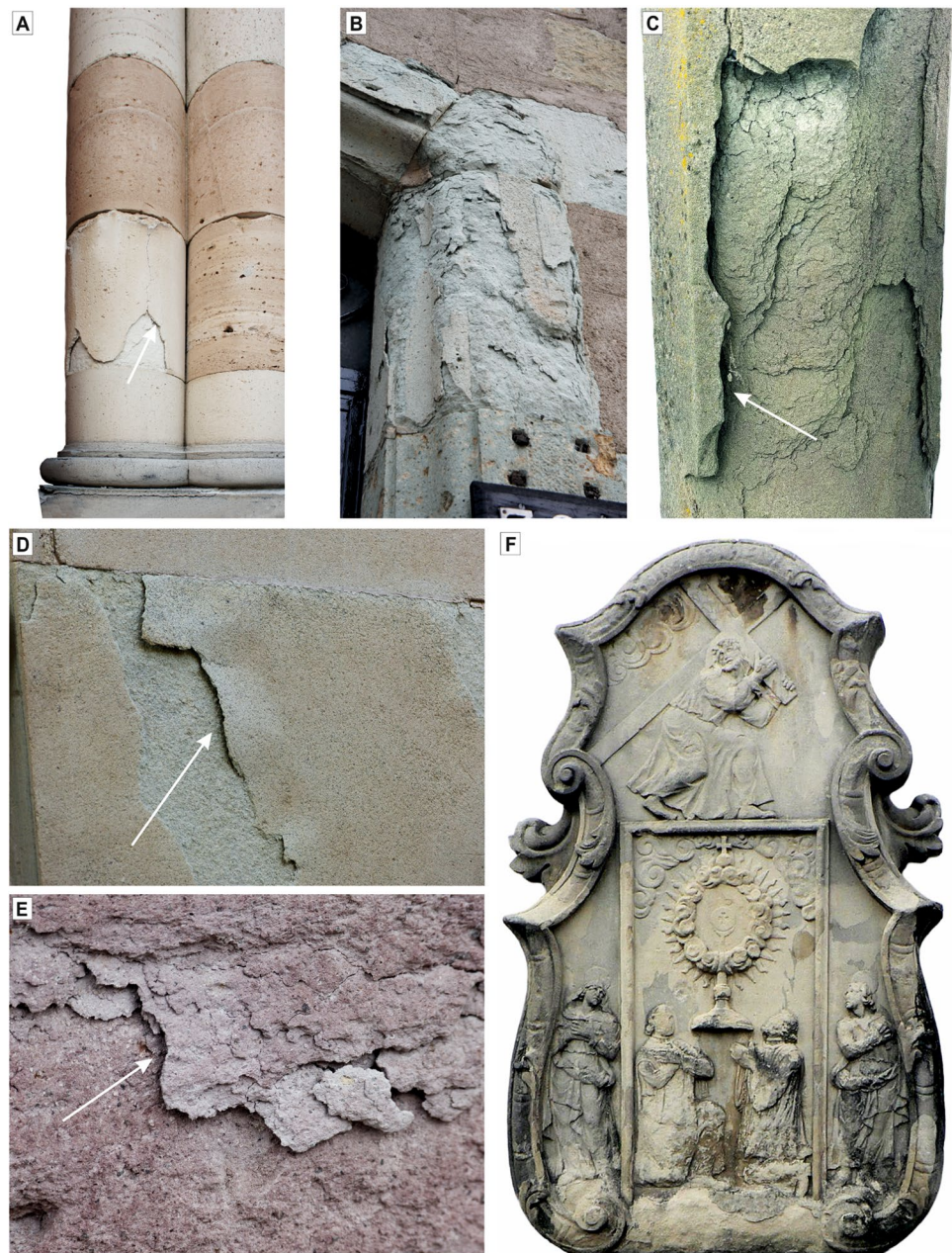
Fig. 2 Exemplary damage features in some of the investigated tuffs and sandstones. A Columns constructed from Blanca Pachuca tuff showing layer-parallel peeling of the stone (white arrow). B extensive flaking damage of Cantera Verde used for doorway lintels similar to the Armenian Blue Sevan tuff, C massive damage (white arrow) to the Schleerieth sandstone which lacks swellable clay minerals, D close-up of scaling damage in the Loseros tuff, E example of the type scaling into rock fragments in the Mexican Cantera Rosa tuff, and F detail of the weathering damage in the Baumberger calcareous sandstone
