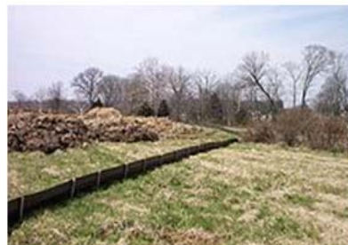
Fig. 17: Silt fence installed on a construction site, ( http://en.wikipedia.org/wiki/file:silt_fence.jpg )
