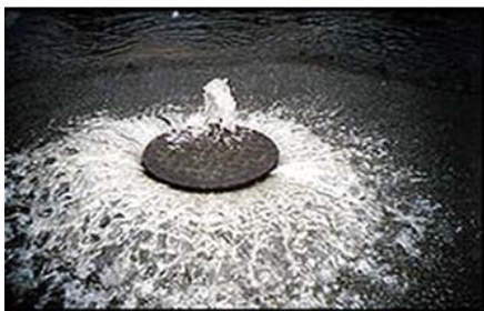
Fig. 7: A manhole cover unable to contain a sanitary sewer overflow, ( http://en.wikipedia.org/wiki/file:sewer-overflow-ri-epa.jpg )
