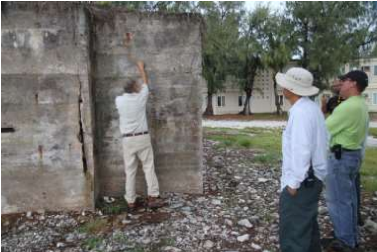
Robert Lodge demonstrating to BOS personnel how to locate voids that need grout injection and/or pinning.
