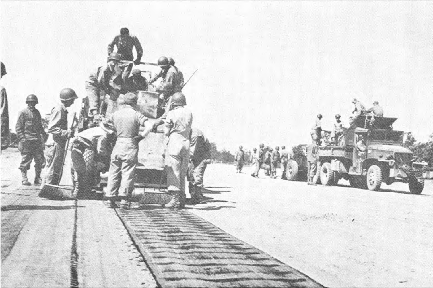
AIRFIELD CONSTRUCTION: HESSIAN MAT
