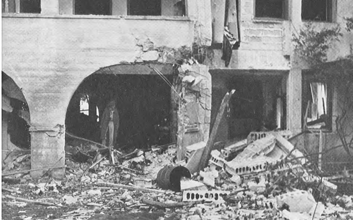
DAMAGE TO BARRACKS, WHEELER FIELD
