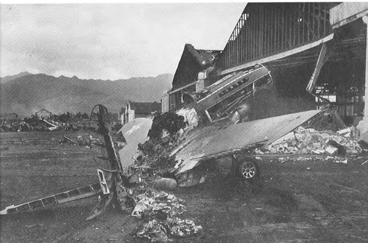
DAMAGE AT WHEELER FIELD
