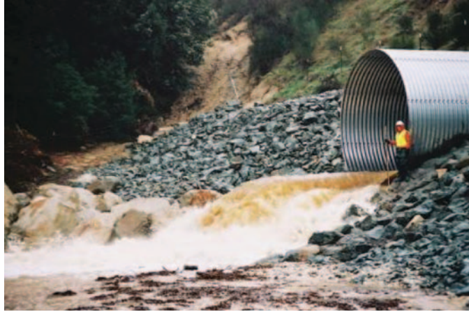
Figure 4-1. Culverts of less than 20 feet in span are routinely inspected in many states ( http://www2.dot.ca.gov/hq/oppd/dib/dib83-01-4.htm ).
