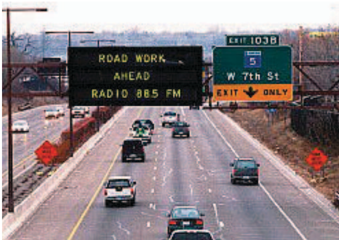
Figure 4-4. Traffic signs include sheeting, posts, and support structures ( http://ops.fhwa.dot.gov/publications/manag_demand_tis/travelinfo.htm ).
