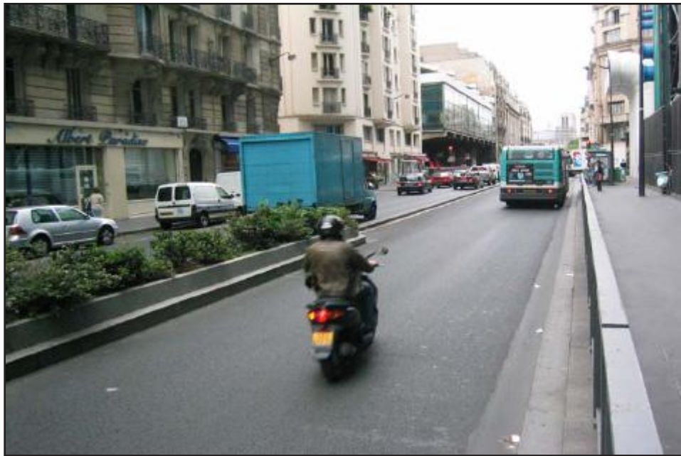
Figure 18. Bus Lane with a Raised Curb and Planter Separating Buses from the Regular Traffic Lane (Paris)
