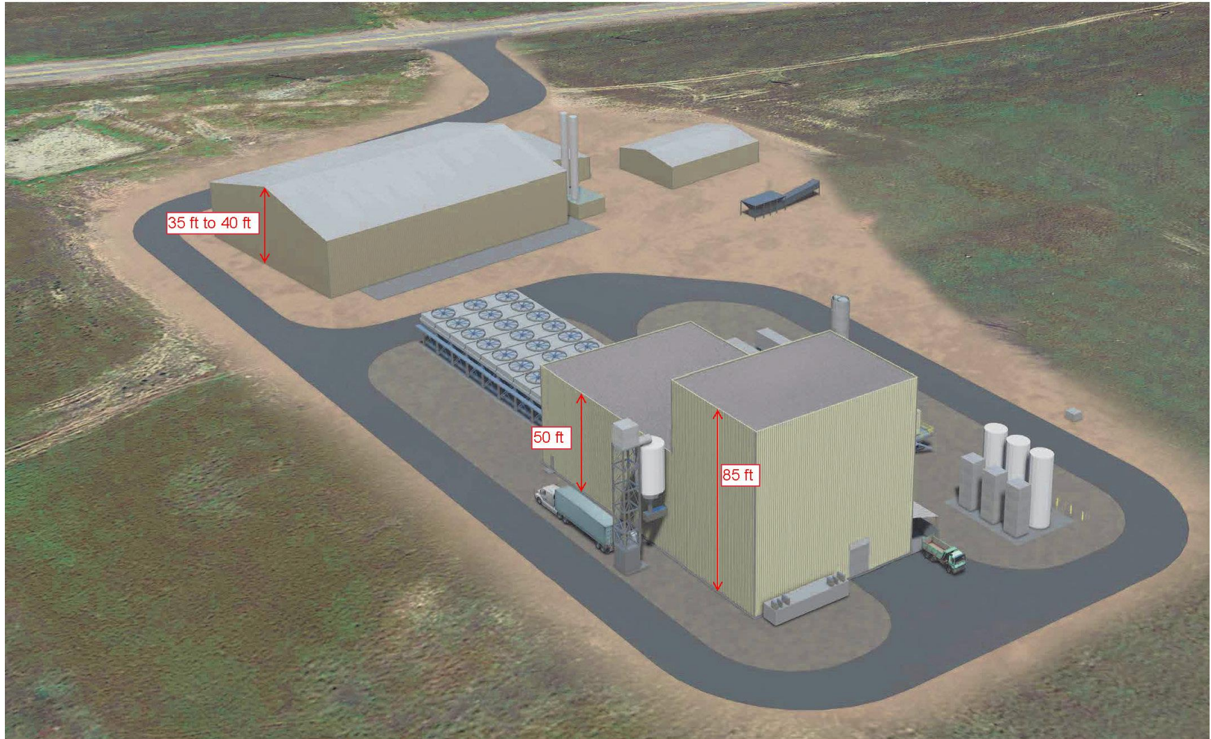
Figure 8 FPO Pilot Site Building Heights
