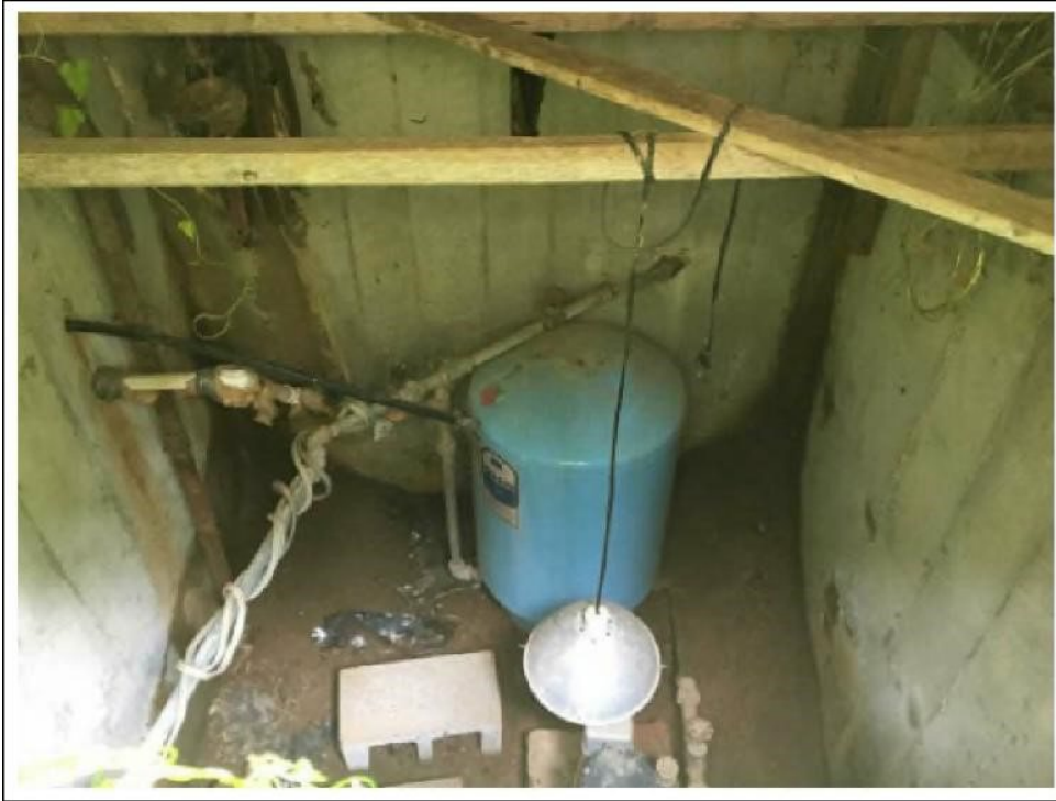
Figure 29. Interior View of H-1 Pumphouse
