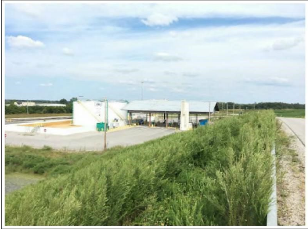
Figure 9. Northeast Facing CSX Facility
