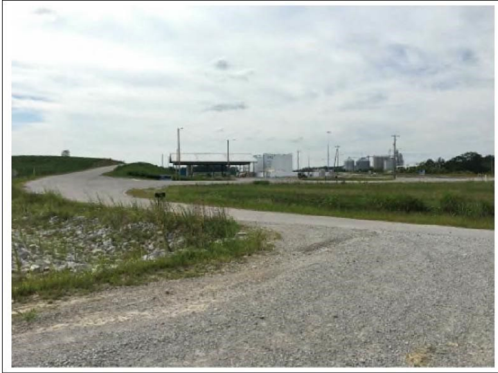
Figure 10. Southwest Facing CSX Facility
