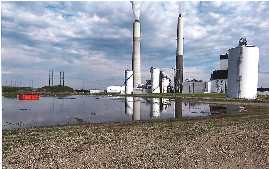
Figure 3 – Proposed Project Site – Ground-level View of Proposed Injection Well Location
