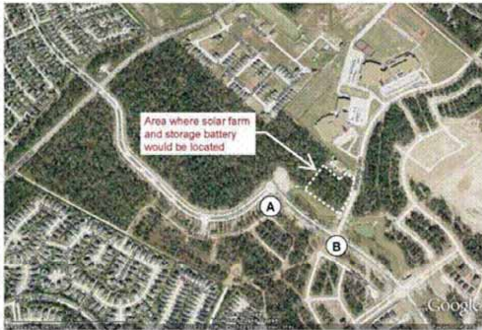
Figure 6. Aerial view of the solar farm and storage battery area. Point A is shown in Figure 7 and Point B is shown in Figure 8.
