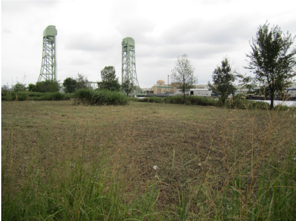
6. Southeastern part of the Project Site
