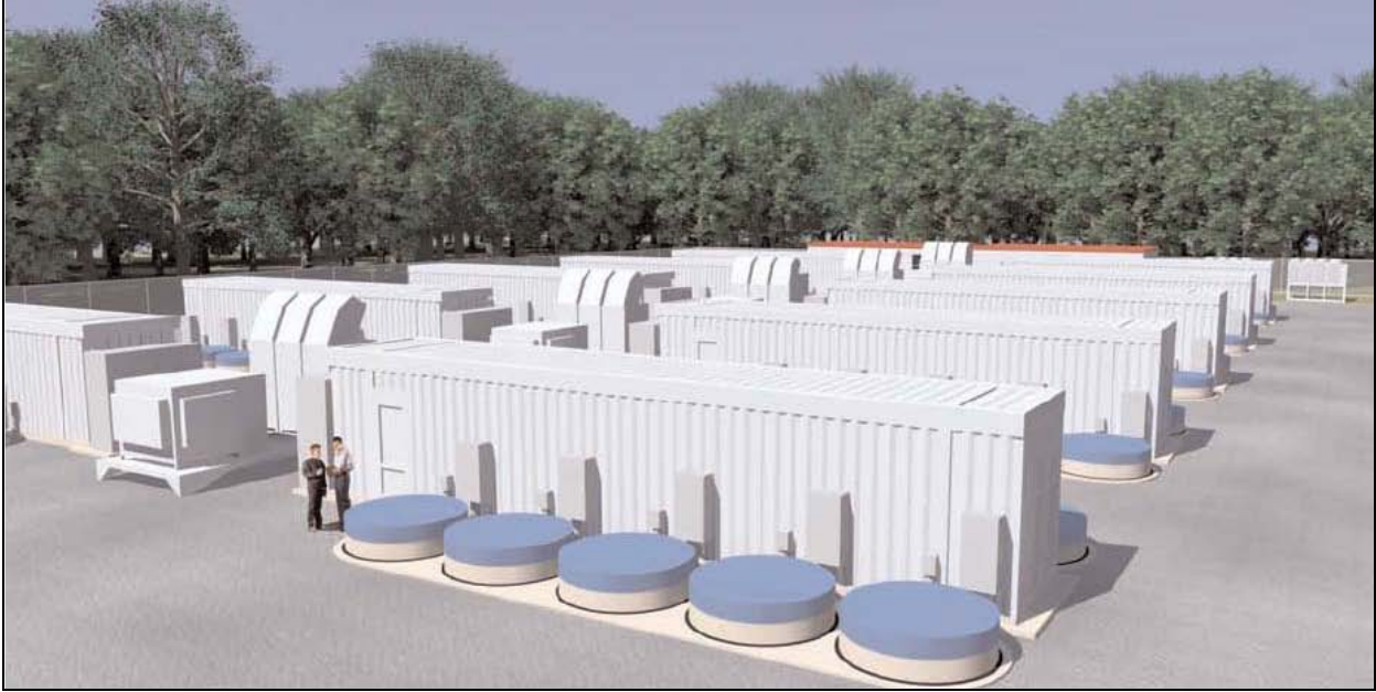
Figure 2-5. Array of 1-megawatt frequency regulation pods.
