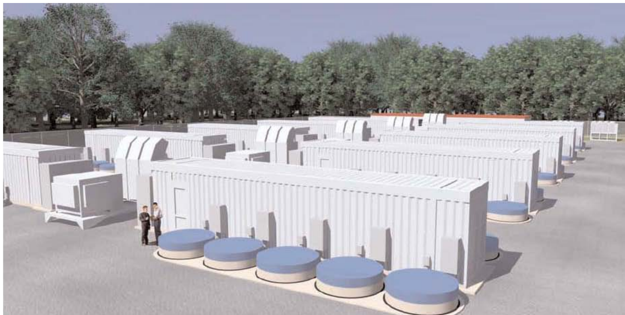
Figure 2-4. Array of 1-megawatt frequency regulation pods.
