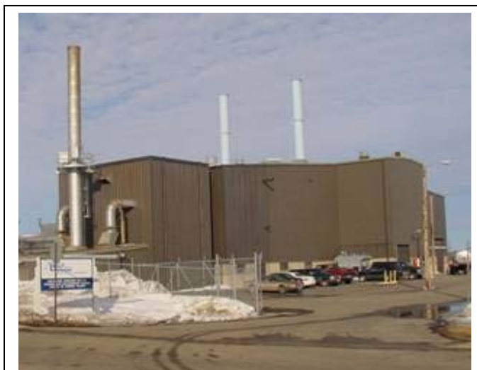
Figure 1-1. PDSWM Waste-to-Energy Facility
