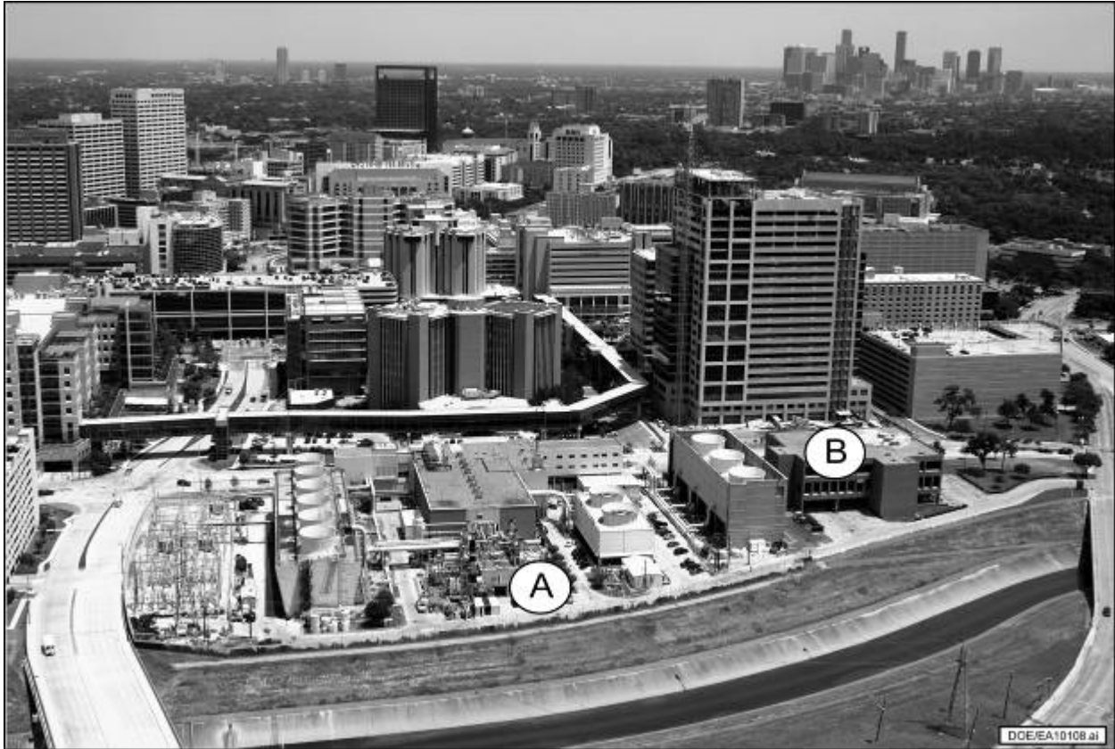
Figure 2-2. The TECO Central Plant prior to expansion and upgrades (view to north). TECO would install the CHP system near the southern boundary of the facility (A) and the four new water chillers in a building being constructed where the laundry facility (B) is shown in this photograph.
