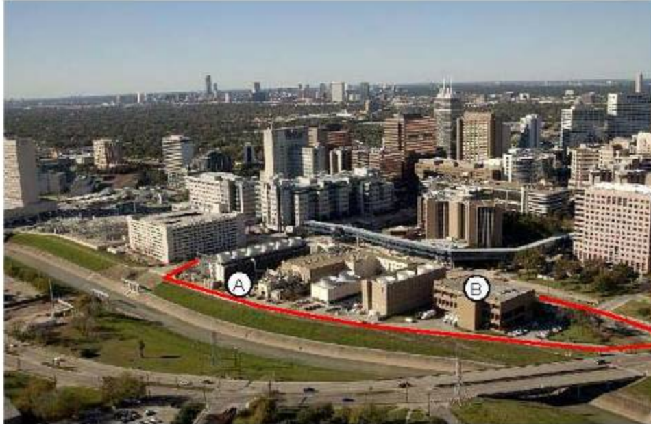
Figure 3. Thermal Energy Corporation Central Plant (outlined in red) (view to northwest). The CHP gas turbine and heat recovery steam generator will be installed near the southern boundary of the property (A). The chillers will be installed in a building currently being constructed on eastern portion of the property (B), where the recently removed Texas Medical Center laundry is shown in this photograph.
