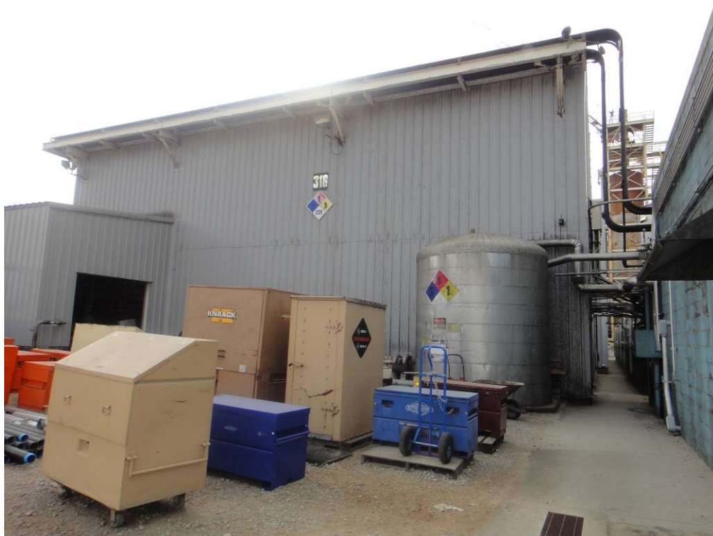
Figure 5. Rear Exterior View of Blower Building
