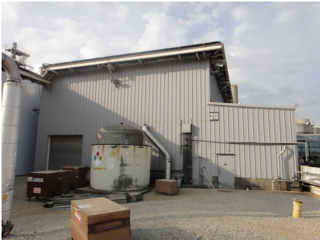
Figure 4. Side Exterior View of Blower Building
