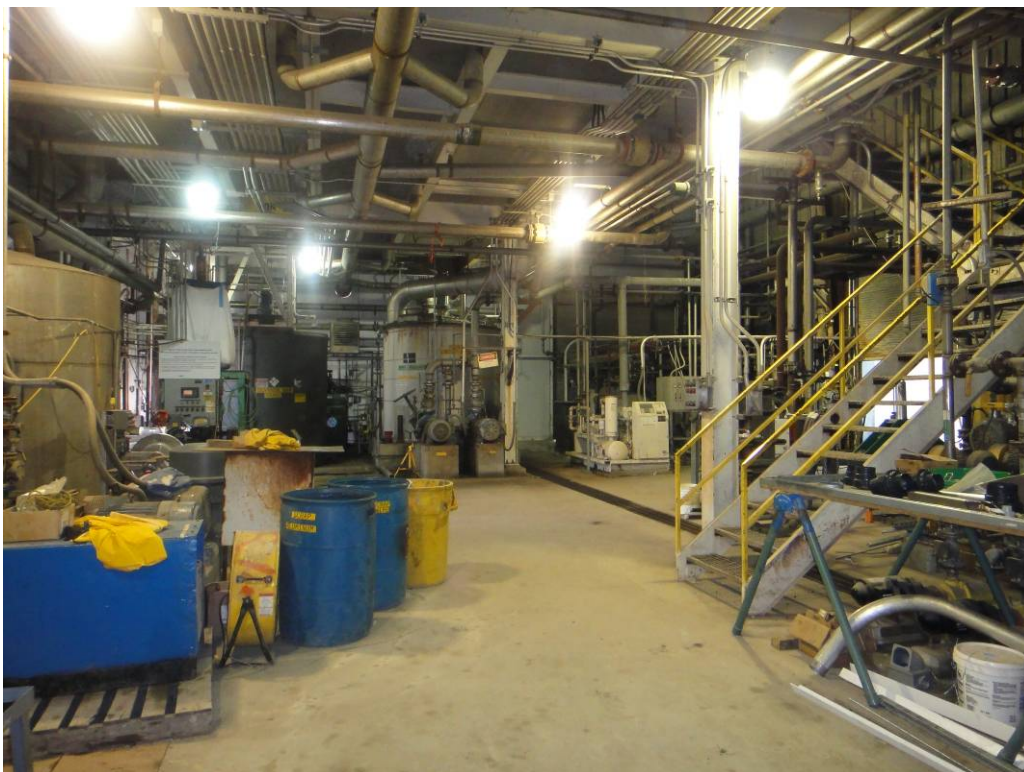
Figure 6. First Interior View of Blower Building
