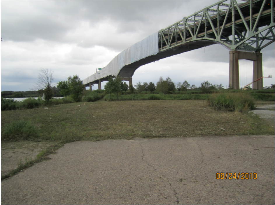
5. Southwestern part of the Project Site
