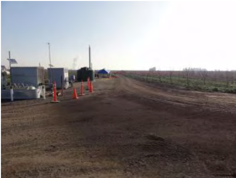
Photograph 4. TFS pad and access road. Photograph taken April 3, 2013.
