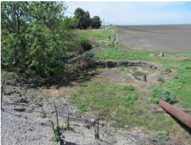
Photograph 8. Irrigation ditch and drainage located at the western pull location and work area at the intersection of King Island Road and Eight Mile Road. Photograph taken April 3, 2013.
