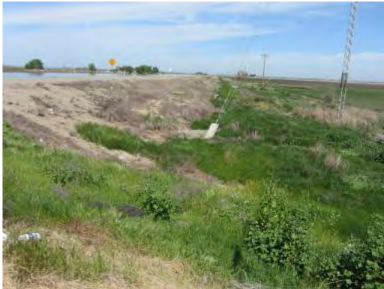
Photograph 10. Eastern pull location and work area at the intersection of King Island Road and Eight Mile Road. Photograph taken April 3, 2013.
