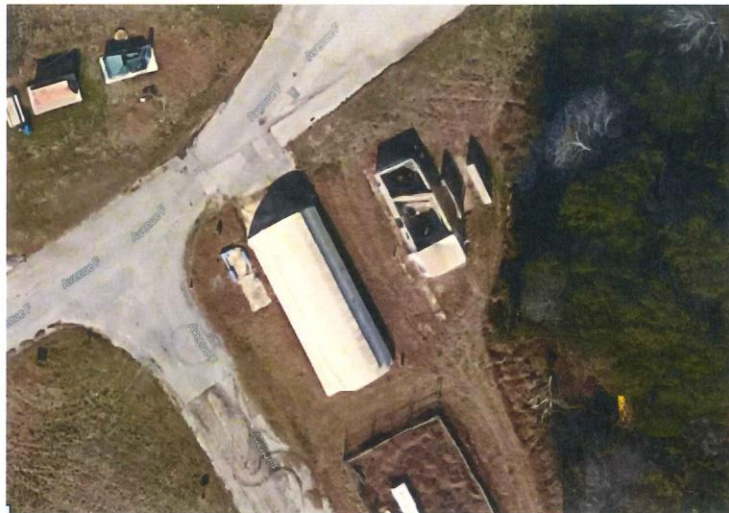
Present imagery (2016) showing Quonset hut building and concrete block structure to the southwest of project site from Google Maps.
