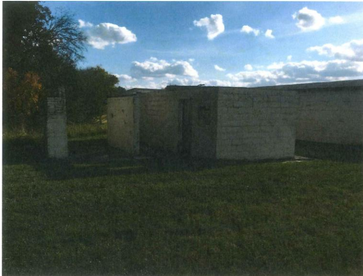
4. View of concrete block structure, facing south.
