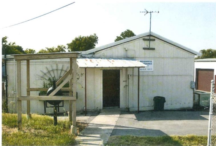
2. View of Building 112 facing south.
