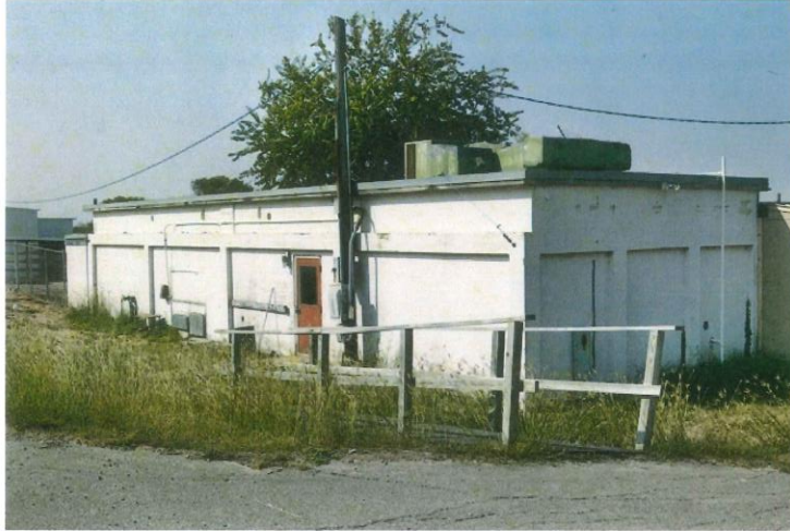
1. View of Building 91, facing south.
