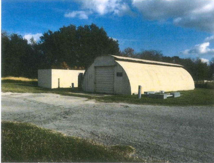
3. View of concrete block structure and Quonset hut, facing southeast.
