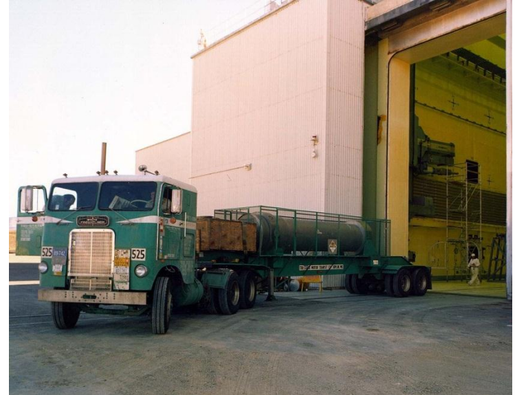
Transportation of Spent Fuel at EMAD
