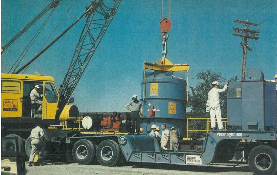
NERVA nuclear reactor and controls were assembled at the Large, PA, Westinghouse Astronuclear Lab, made safe for travel and possible accidents with poison wires, and shipped as one unit to the Jackass Flats, Nevada Test Site (Aerospace America, June 1989).
