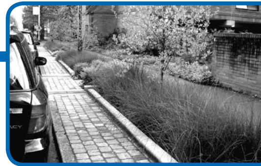
These street planters on SW 12th Avenue on the Portland State University Campus were designed to capture and infiltrate approximately 8,000 square feet of street runoff while still maintaining strong pedestrian circulation and on-street parking in a completely built-out urban environment.
