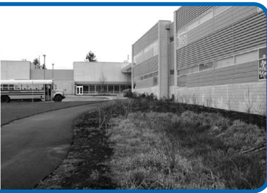
This rain garden at Aloha Huber Park Elementary School treats rainwater collected on the building's roof. Schools are excellent demonstration sites for rain gardens, which can provide hands-on learning opportunities for students.
