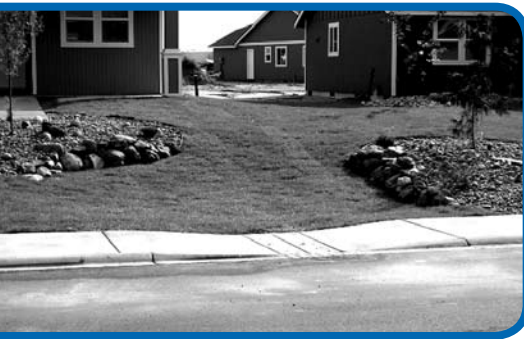
Shallow, grassy swales like this one can be found in new neighborhoods in the City of Boardman, in eastern Oregon. They capture water from the street and the residence on a right of way that is designed to be indistinguishable from the front lawn. The sidewalks are angled to drain toward the swale, away from the street.
