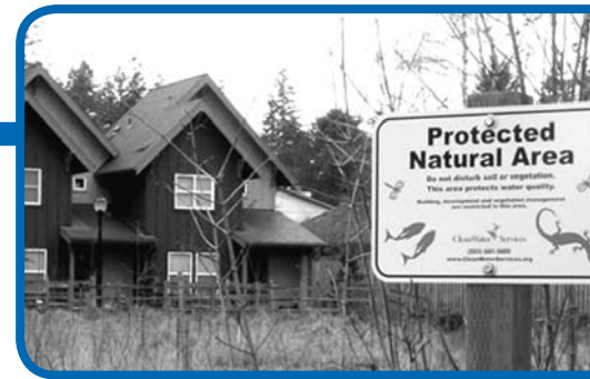
Oleson Woods is a multifamily complex in Washington County owned by Community Partners for Affordable Housing. The site was designed to preserve its mature Oregon White Oaks and Ponderosa Pines, as well as some wetlands.
