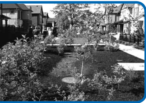
A rain garden at Villebois, a 500-acre community currently under construction in Wilsonville
