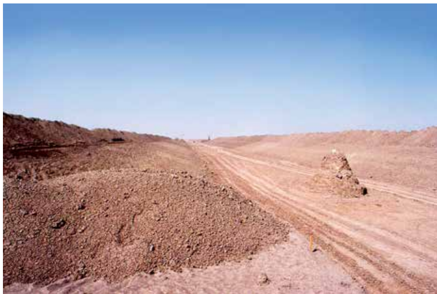
FIGURE 13.2. Photograph of third river drain looking north. (Photo: TJW)
