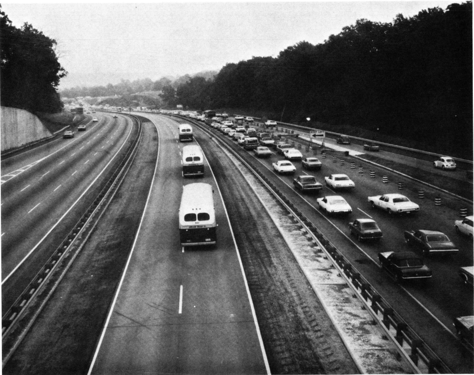
Figure B-61. Completed section with reversible bus lanes, Shirley Highway, Virginia.
