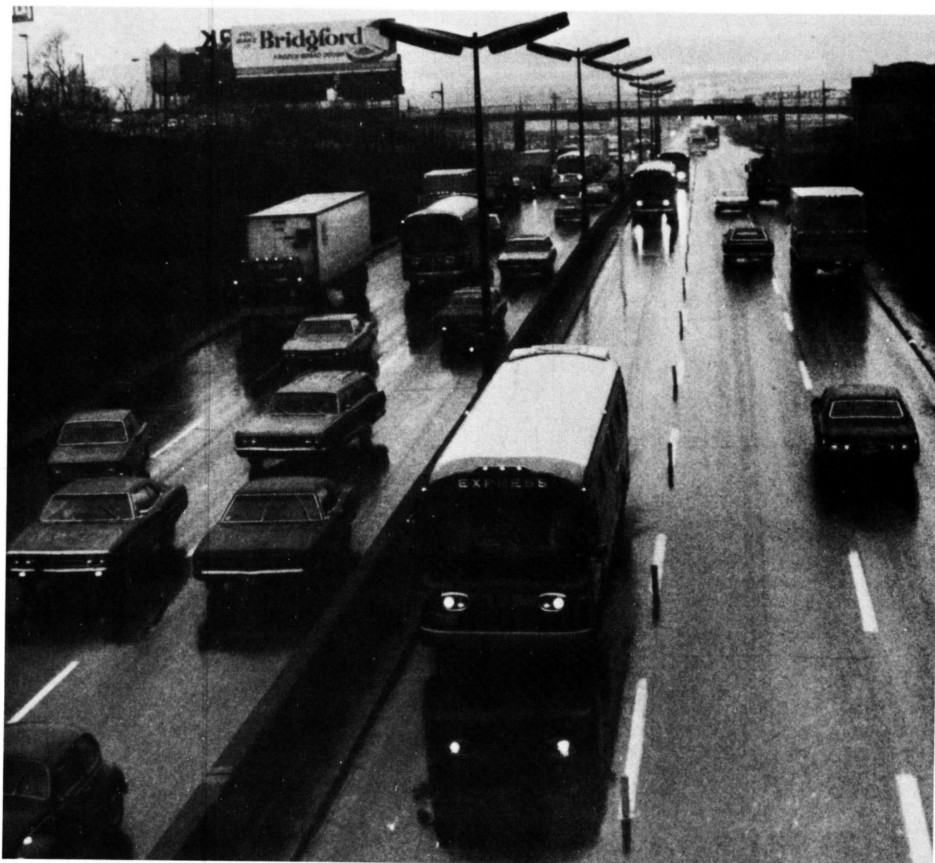
Figure B-29. Typical view, I-495 exclusive (contra-flow) bus lane, New Jersey.
