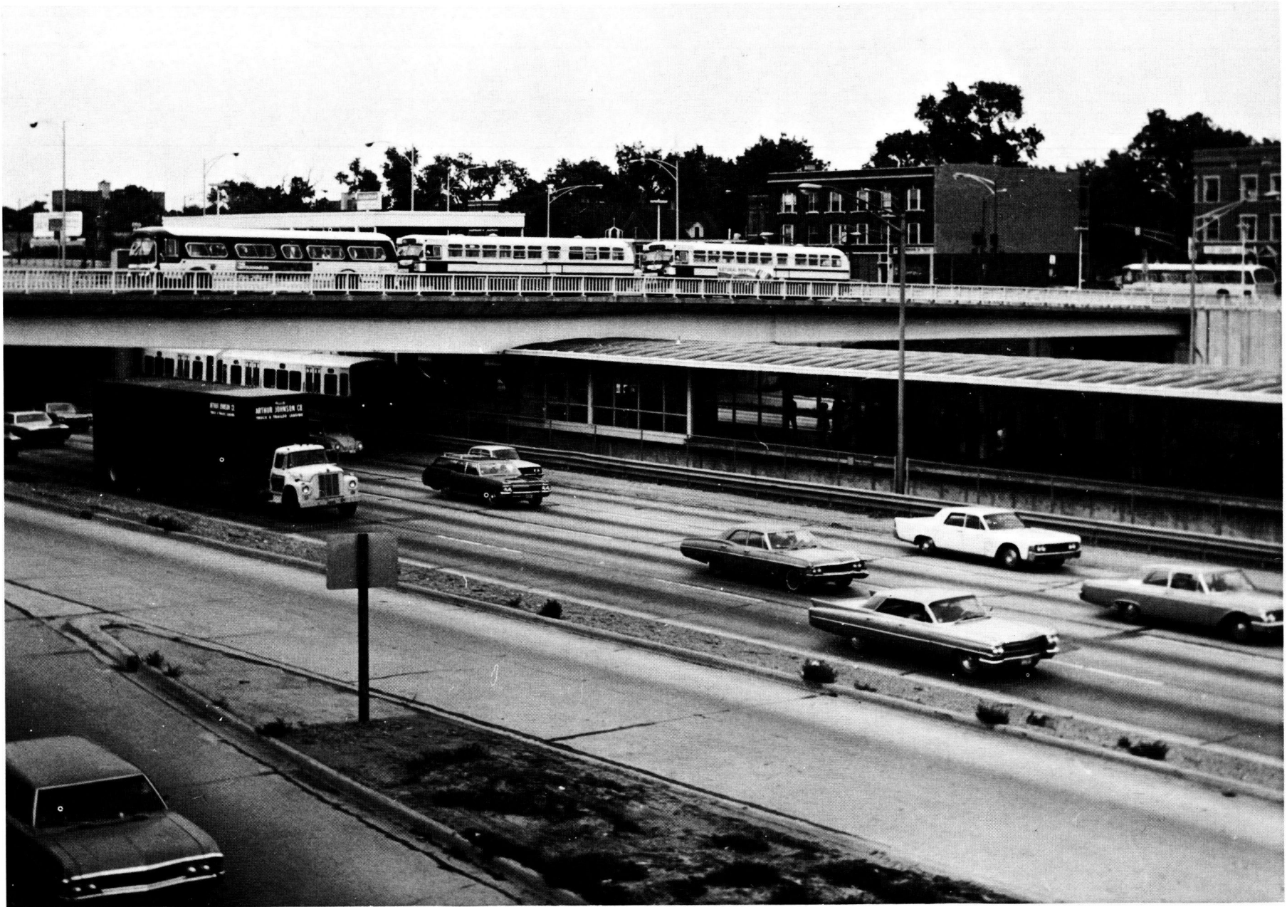
Figure D-5. 69th Street-Dan Ryan Expressway bus bridge and terminal, Chicago, Ill.
