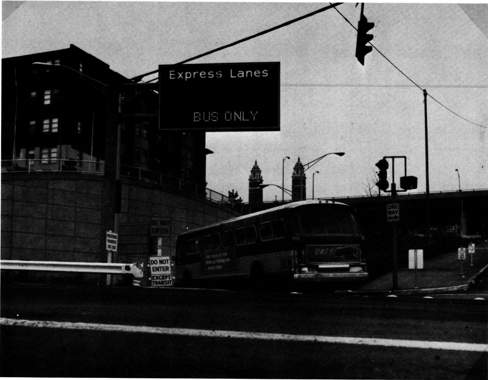
Figure B-56. Blue Streak exclusive northbound bus ramp onto I-5, Seattle, Wash.
