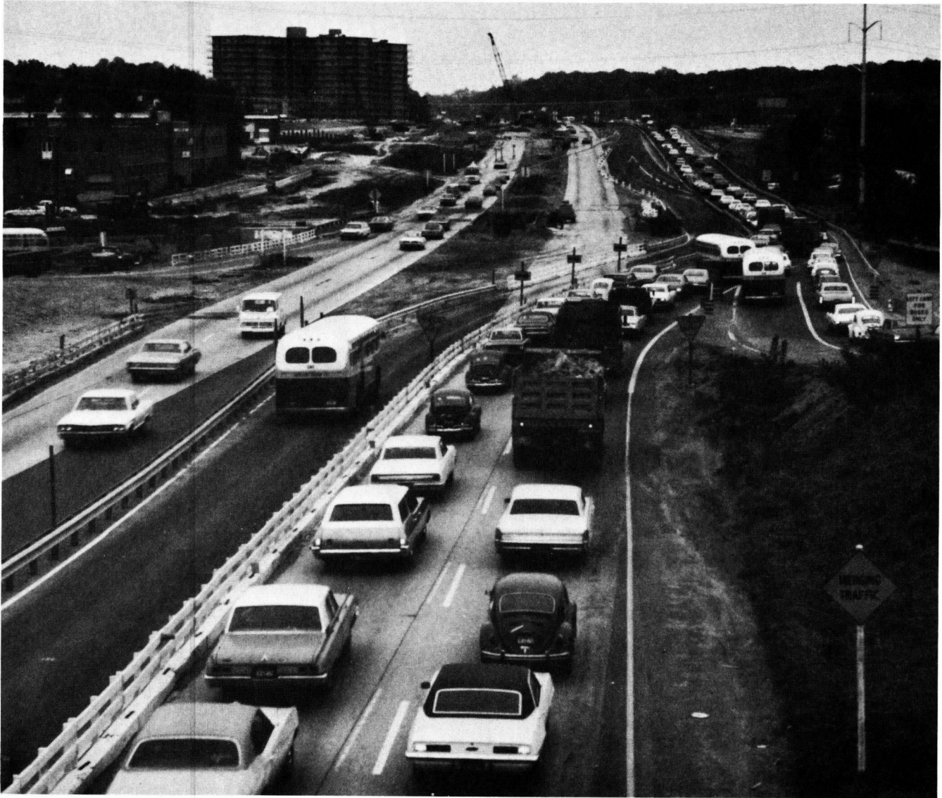
Figure B-64. Bus access to temporary bus lane (looking north from Shirlington Circle), Shirley Highway, Virginia.
