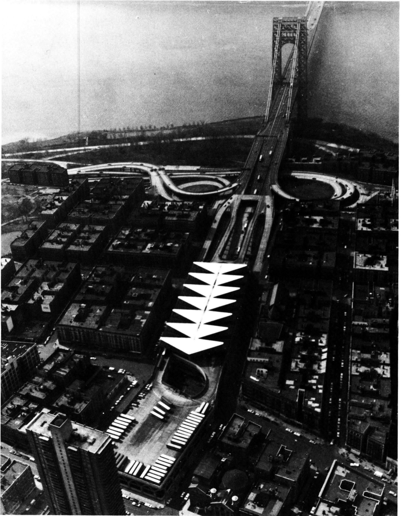
Figure D-15. George Washington Bridge Bus Terminal, New York City.
