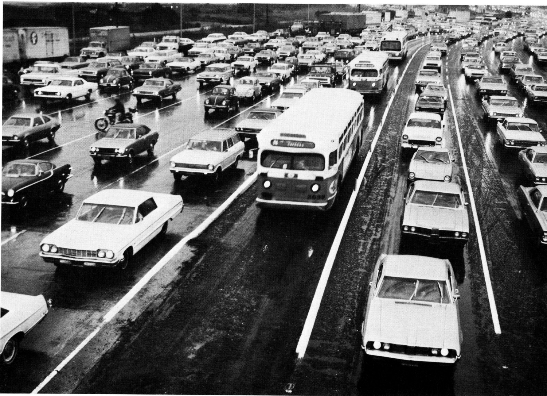
Figure B-47B. Bus bypass of car queues at toll plaza, San Francisco-Oakland Bay Bridge.
