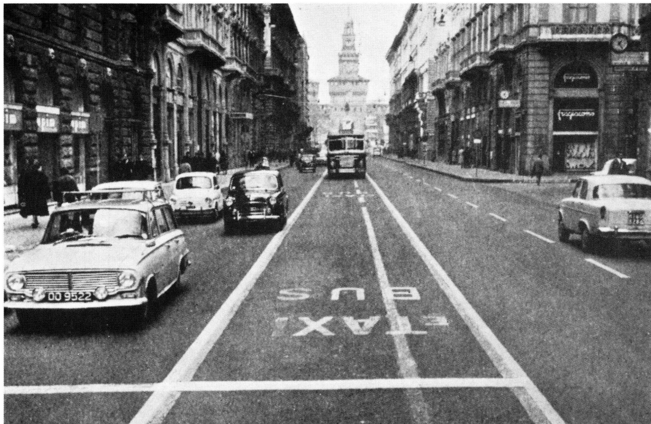
Figure C-80. Via Dante median bus lane, Milan, Italy.
