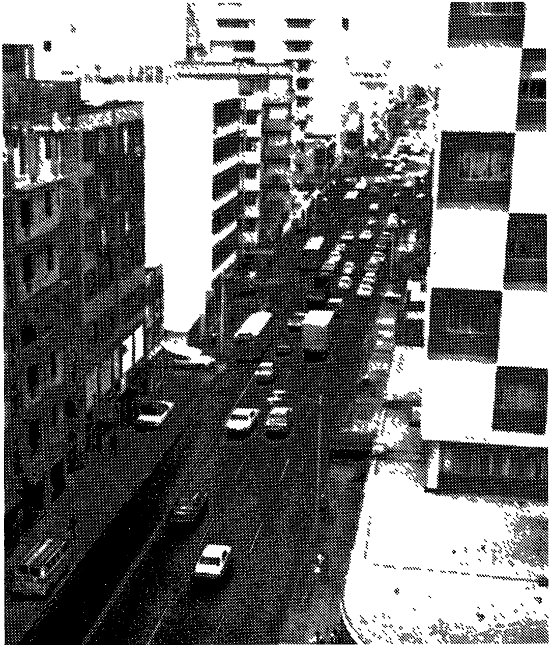
Figure C-48 Typical view, Avenida Ponce de Leon contra-flow bus lane, San Juan, P R
