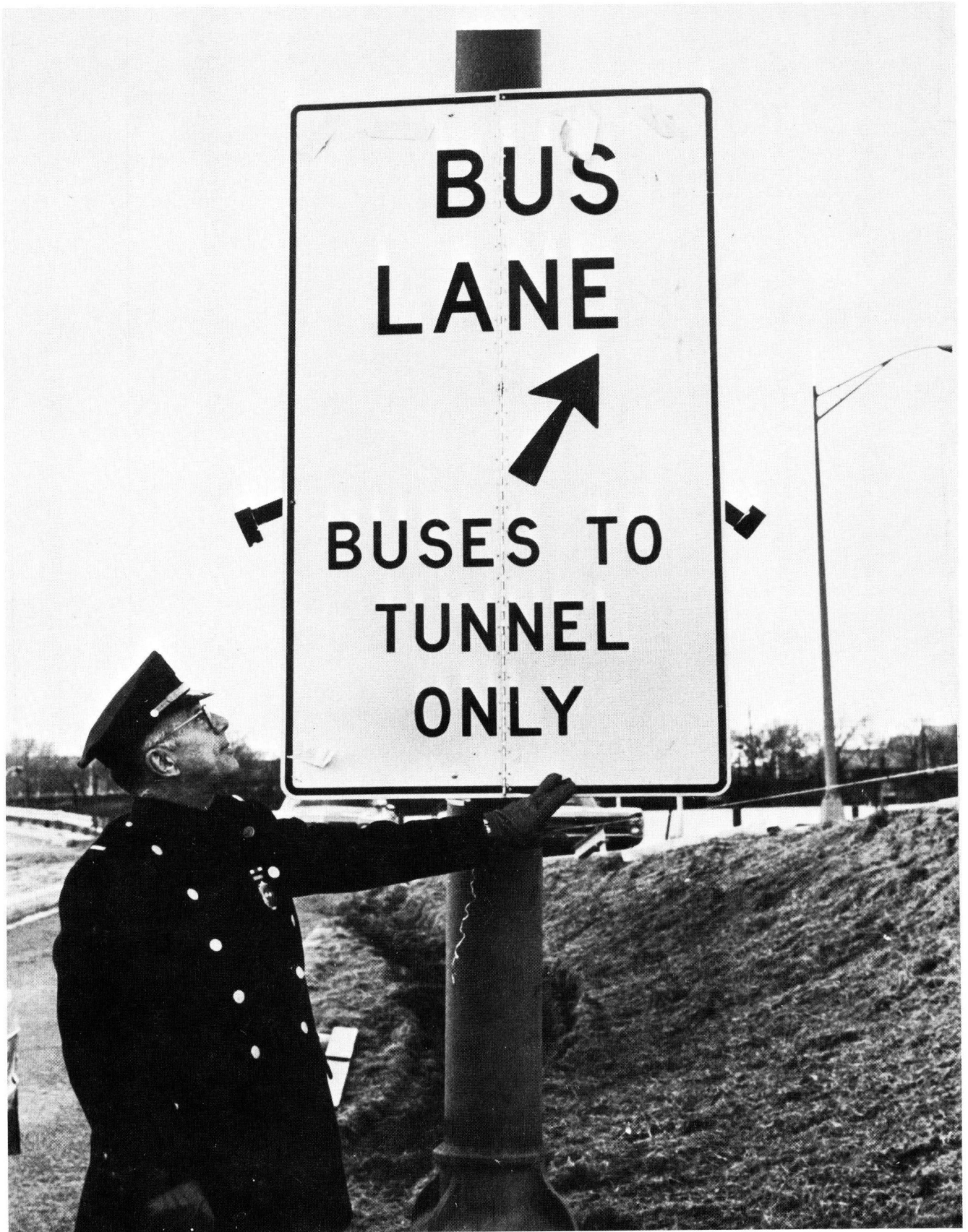
Figure B-32. Typical hinged sign, I-495 exclusive (contra-flow) bus lane, New Jersey.
