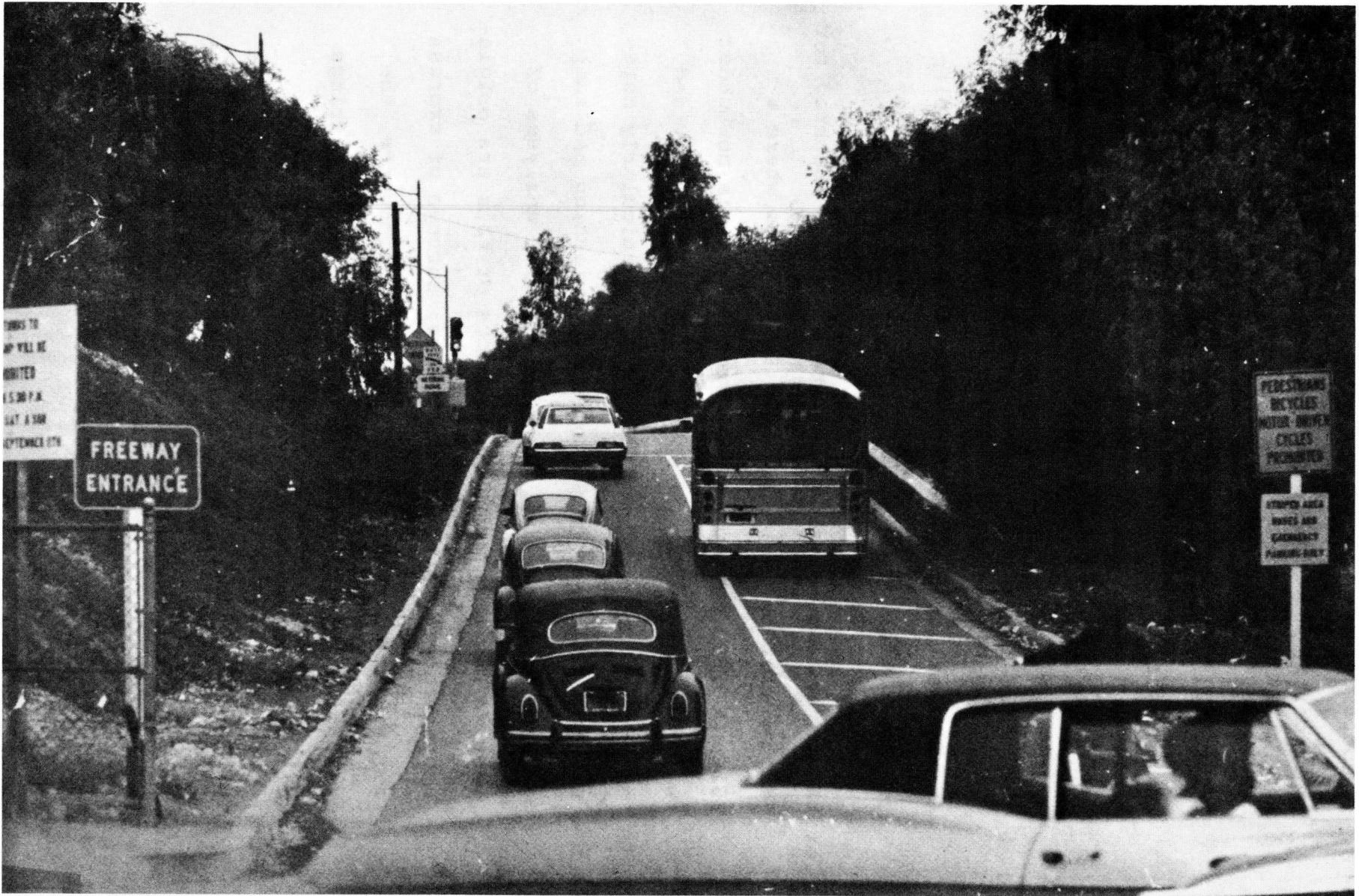
Figure B-16. Example of bus priority treatment at metered freeway ramps, Los Angeles, Calif.
