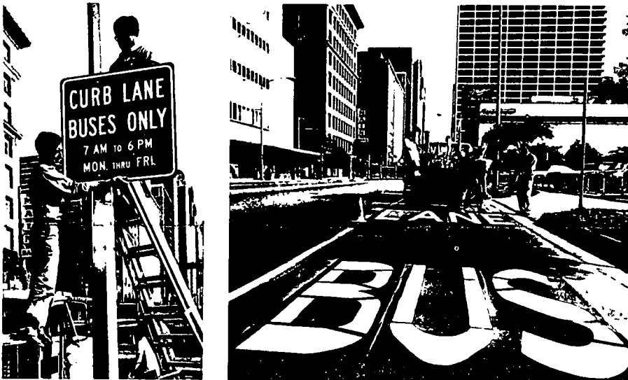
Figure C-26. Signs and markings, Main Street bus lane, Houston, Tex
