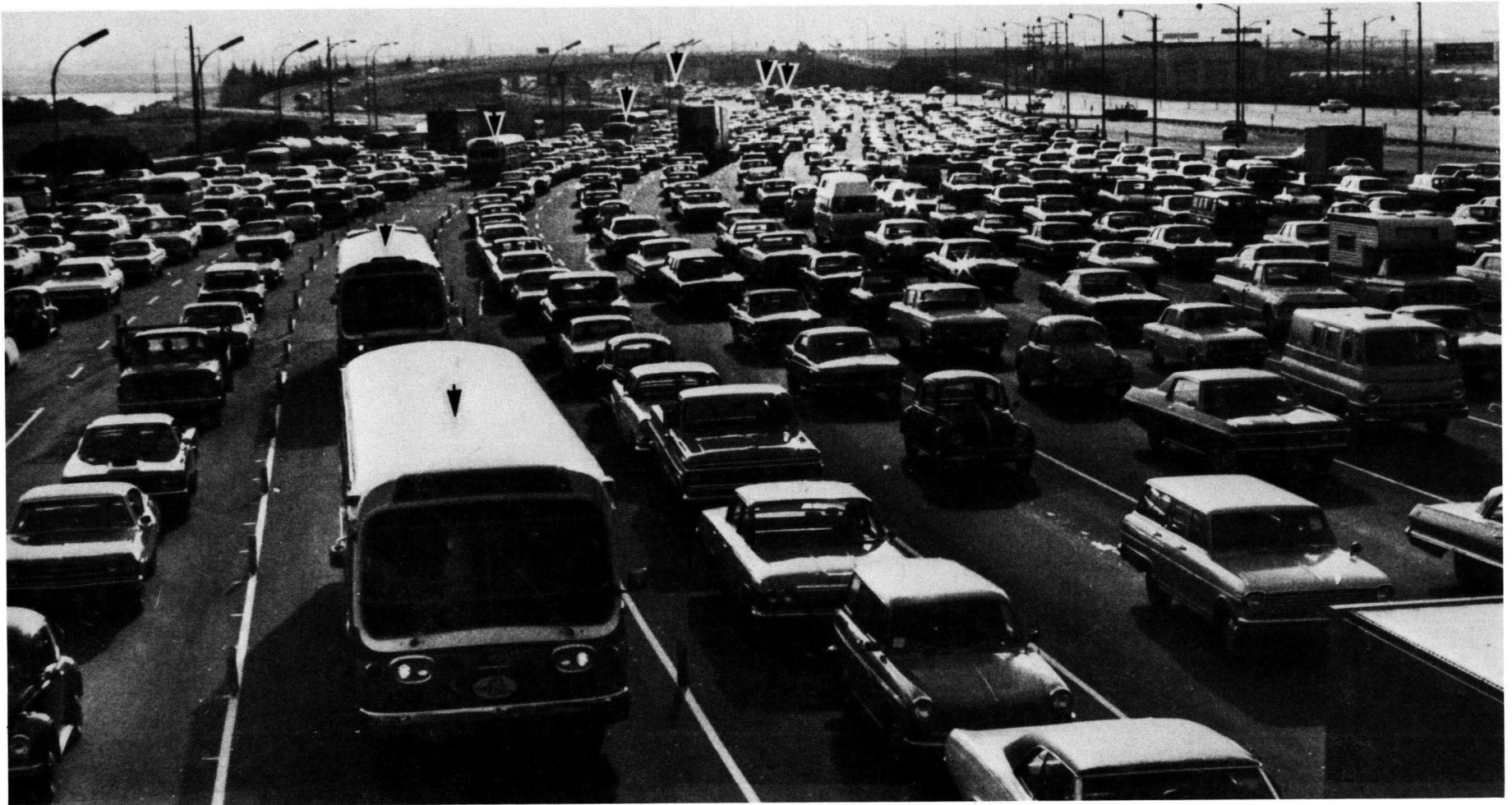
Figure B-47C. Bus bypass of car queues at toll plaza, San Francisco-Oakland Bay Bridge.
