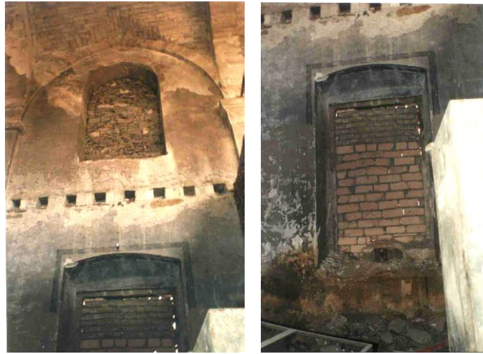
Figure 3.6 View of beam traces of the mezzanine floor and canceled window openings (ÇE-MİM, 2001)
