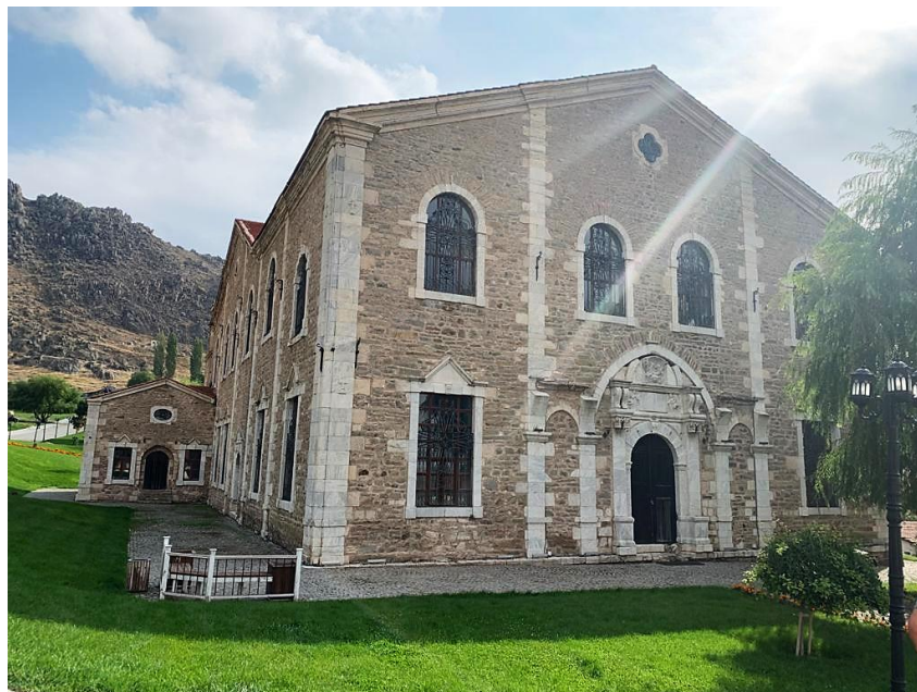
Figure 3.7 Exterior view of Surp Yerrortutyun Church from the western entrance in 2020 (Source: photographed by the author)
