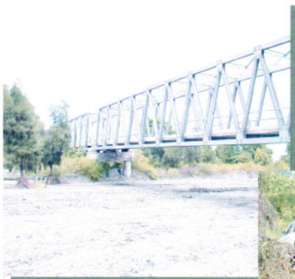
Steel Truss Bridge
