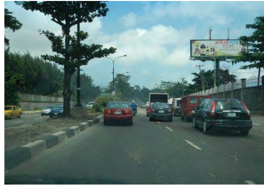
Source: Photographed by Study Team Figure 7-4 Road that requires works to build the Monorail (Ahmadu Bello Way on Victoria Island)
