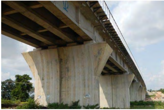
Source: Photographed by Study Team Figure 3-19 Panoramic View of Viaduct
