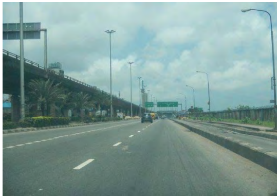
Source: Photographed by Study Team Figure 7-3 Road that has Sufficient Space for Monorail (Ring Road (south coast) on Lagos Island)
