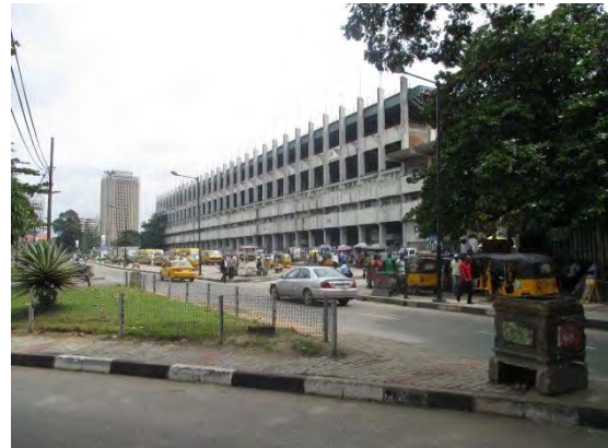
Source: Photographed by Study Team Figure 5-5 Local Road on Lagos Island
