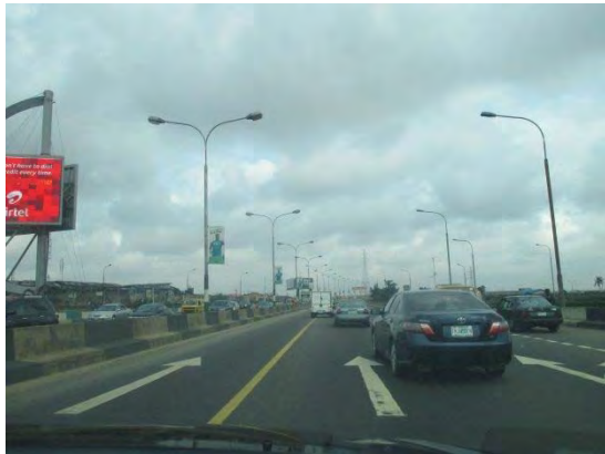
Source: Photographed by Study Team Figure 5-4 Third Mainland Bridge
