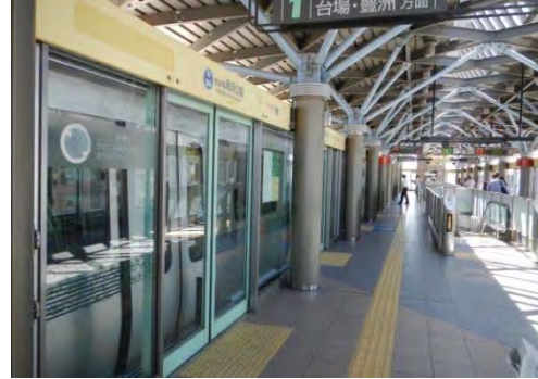
Source: Photographed by Study Team Figure 6-16 Platform Screen Door
