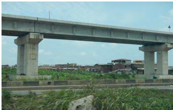
Source: Photographed by Study Team Figure 3-21 Panoramic View of Viaduct
