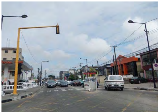
Source: Photographed by Study Team Figure 7-5 Road that requires works to build the Monorail (Awolowo Road on Lagos Island)
