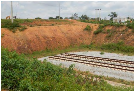
Source: Photographed by Study Team Figure 3-17 Civil Engineering Section (Road Intersection)
