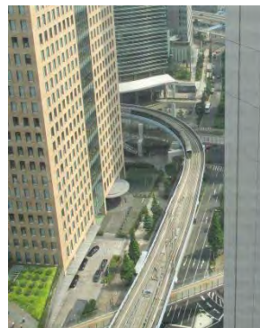
Source: Photographed by Study Team Figure 6-13 AGT Curved Structure
