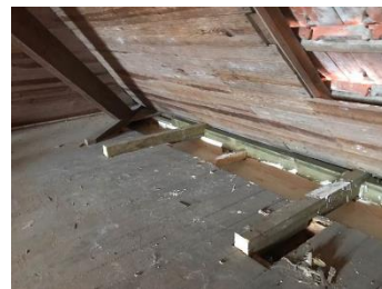
Figure 9. Splice of wooden beams (credits: Aníbal Costa)
