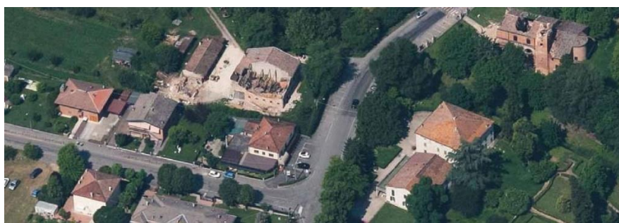
Figure 2. Medolla, Modena. The roof, resting on long span walls, collapsed and directly contributed with its thrust to the out-of-plane overturning of the walls.
