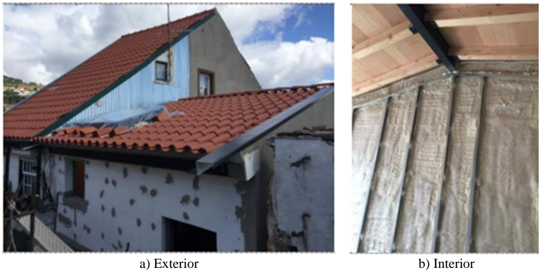
Figure 7. Thermal insulation of walls
