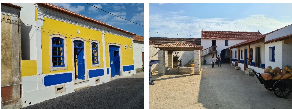
Figura 12. Front façade and the courtyard of the Gandaresa House, Seixo, Mira (credits: Aníbal Costa)
