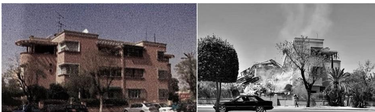
Figure 2. Demolition of a building in Gueliz , the centre of Marrakech , Morocco.
