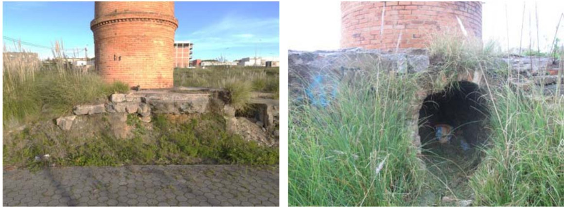
e) Block at the chimney's base
