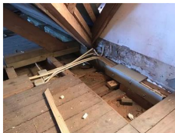
Figure 8. Repair of connections between roof structure with floor beams (credits: Aníbal Costa)
