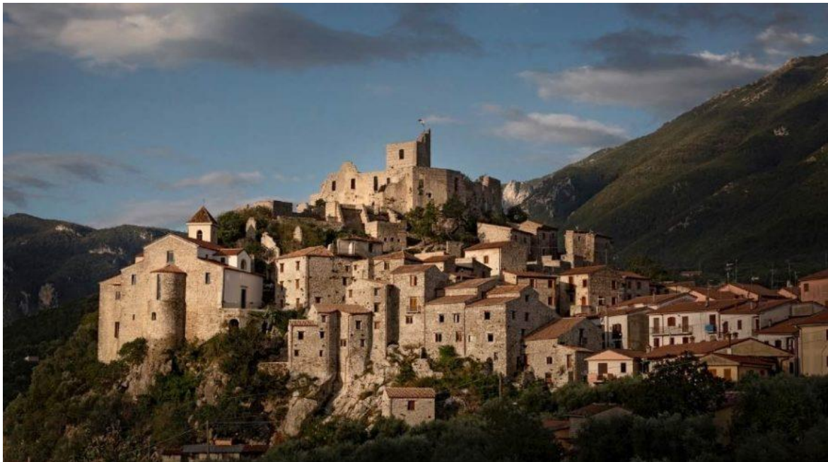
Figure 1. View of the castle and village after restoration work.
