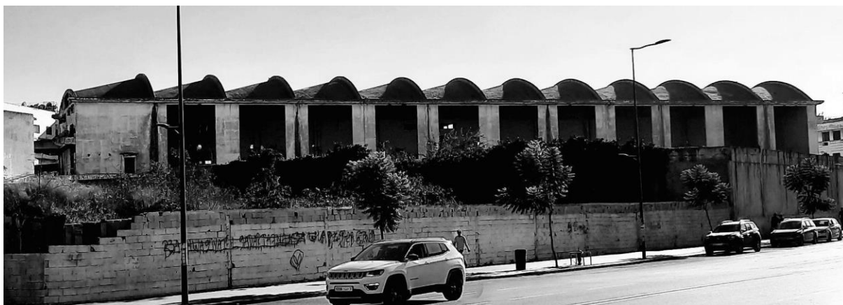
Figure 1. S.I.M, an abandoned industrial enterprise in Roches Noires, Casablanca, Morocco
