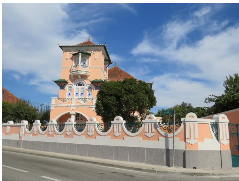
Figure 10. Cestinhos house at the end of minimum intervention (credits: A. Tavares)
