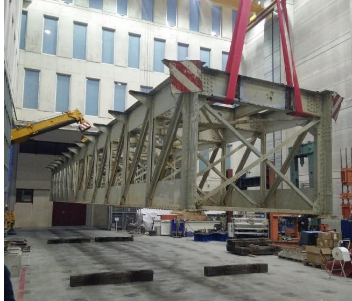
Figure 2. The bridge during its positioning.
