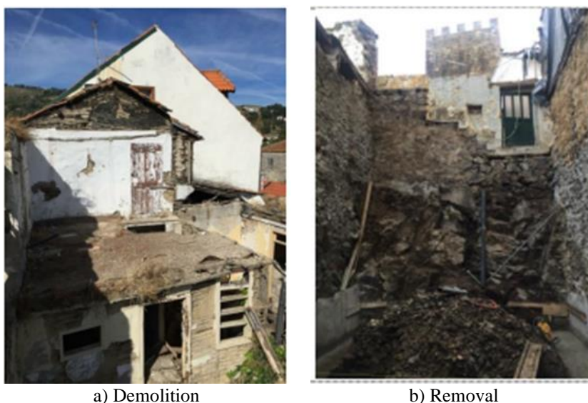
Figure 2. Demolition and removal of the demolition waste
