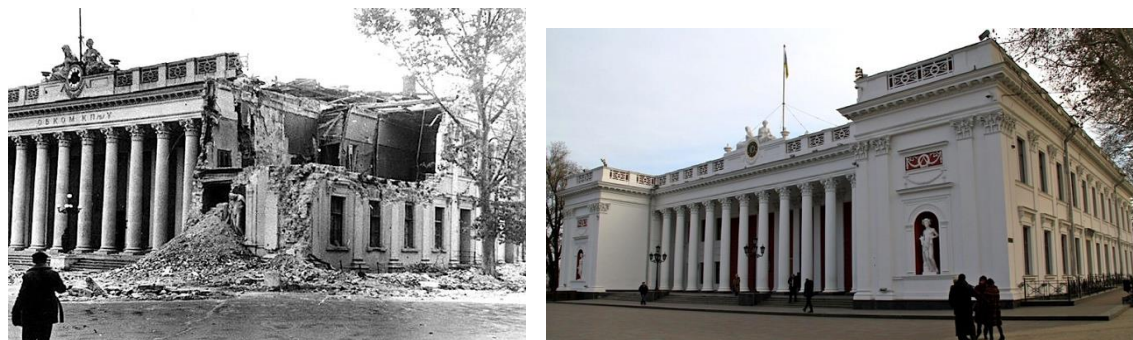
Figure 10. Restoration of the building of the city hall of Odessa, arch. G. Topuz, 1949
