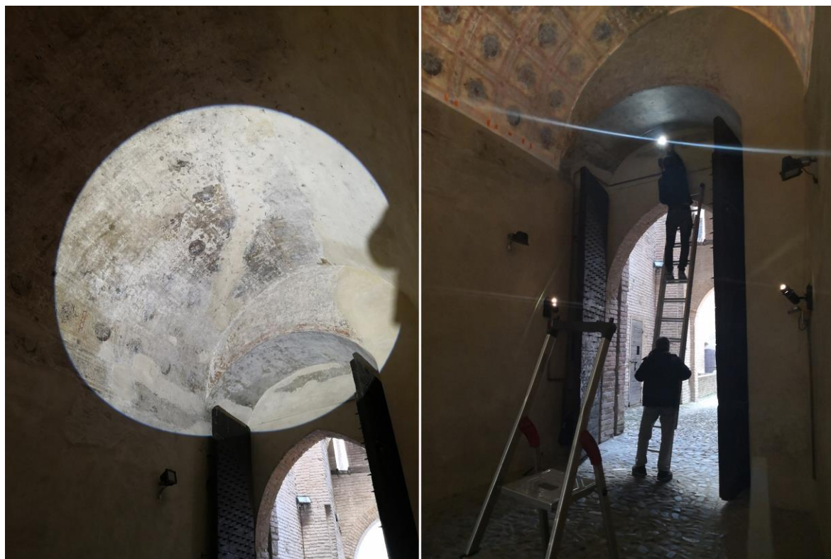
Figure 8. The seven projectors were first fixed in the physical environment of the Rocca and then their necessary position was calculated to set the rendering phase.
