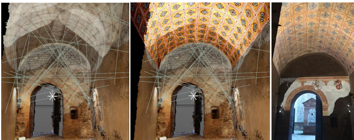
Figure 9. The sequence of geometric operations carried out to determine the definitive projection. Left to right: 3d digital model with cameras placed in the projection points; 3d model mapped with reconstructed texture of lacunars; picture of the final projection on the real vault
