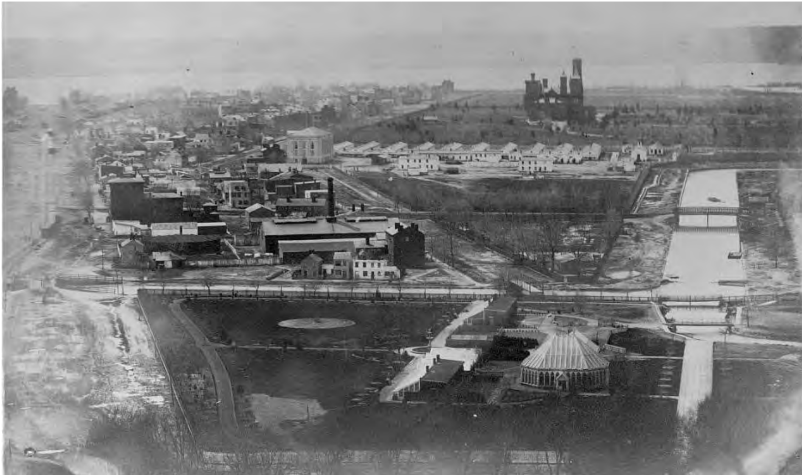
Historic Figure 6 of 10 – As shown in this 1861 photograph from the Capitol, the federal government utilized parts of the Mall for military purposes during the Civil War. The low buildings in front of the Smithsonian Castle were part of the Armory Square hospital complex. Note the presence of the Washington City Canal (opened 1815, converted to sewer ca. 1870) on the right side of the photograph. (Library of Congress)
