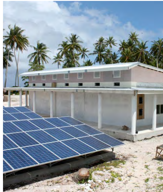
FIGURE 5: BATTERY ROOM ON NUKUNONU.
