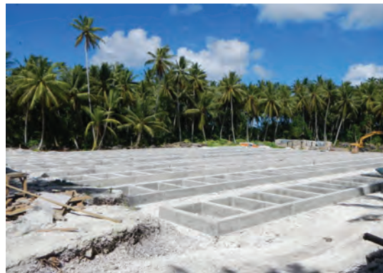
FIGURE 4: THE ARRAY FOUNDATIONS ON ATAFU.
