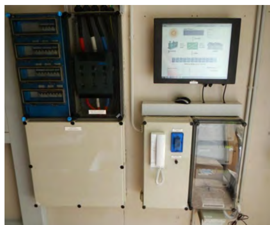
FIGURE 21: THE TOUCHSCREEN COMPUTER AND THE THREE WEBBOXES (TO THE RIGHT OF THE BLUE ALARM, NEXT TO THE PHONE)
