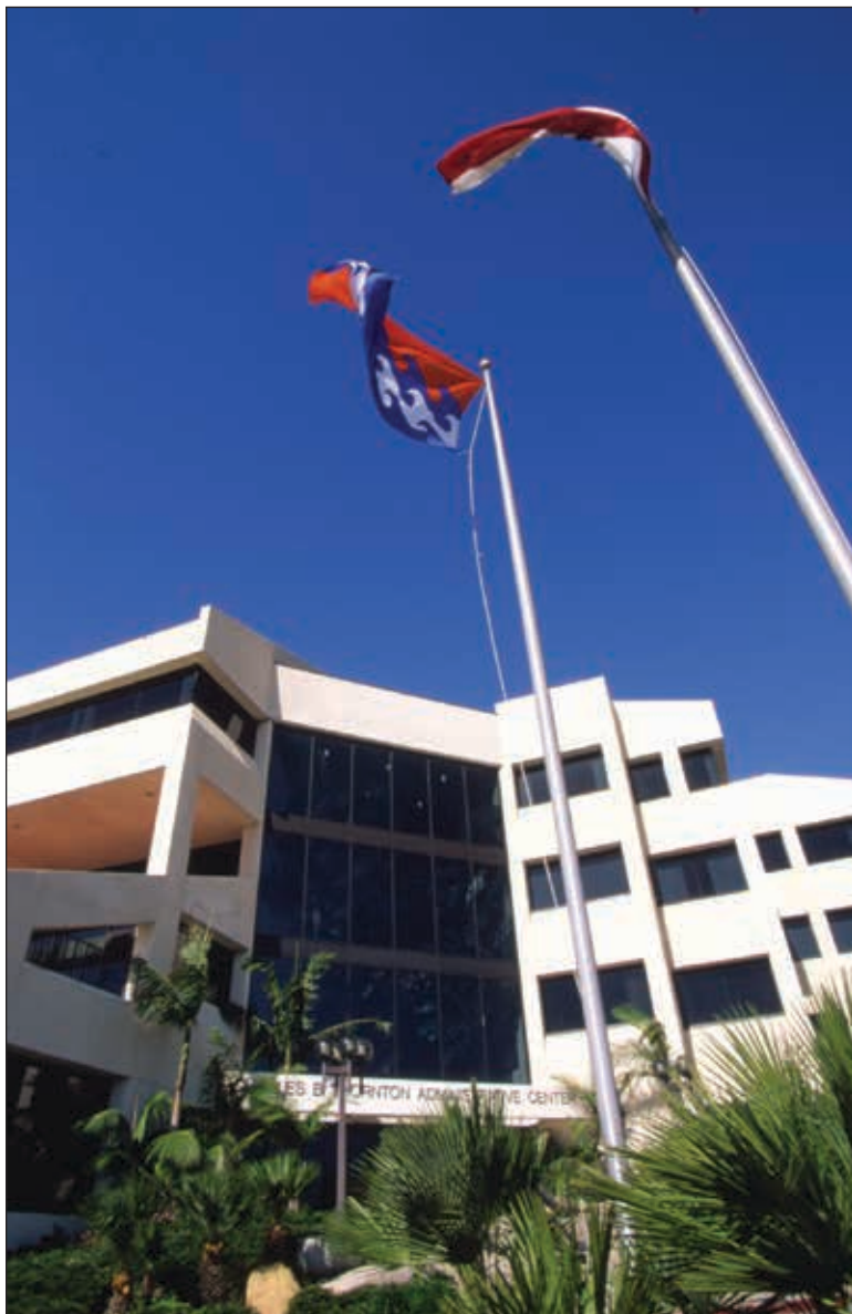
The Thornton Administrative Center houses many University employees and offices including the Office of Student Information and Services.
