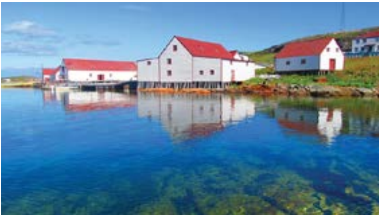
Figure 5.2. Battle Harbour as history in place: the salt store, which was the largest in Labrador, was the most important building on the site because of the value of salt to the traditional fishery. (Photo credit: Mark C.J. Stoddart, 2013)
