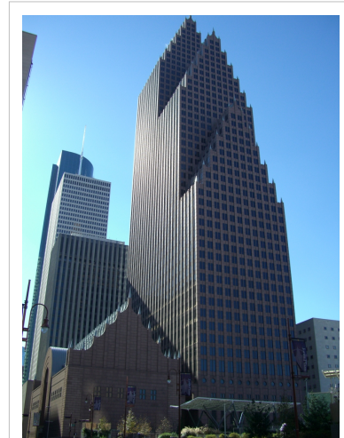
Bank of America Center in Houston by John Burgee and Philip Johnson. It combines architecture elements of pre-WWII skyscrapers with elements of modern aesthetics.
