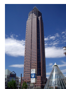
Meseturm in Frankfurt, Germany by Helmut Jahn. Completed 1991.
