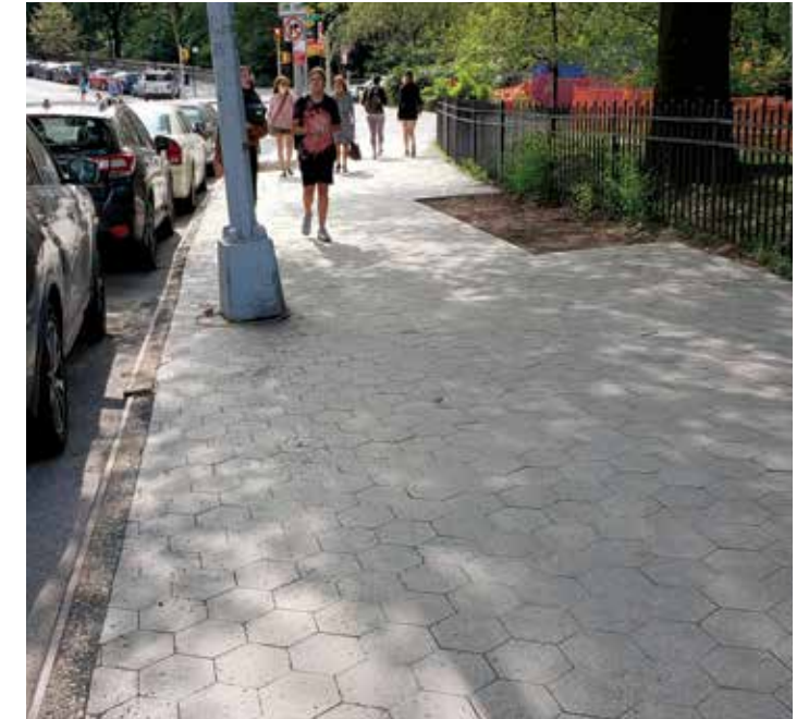
After: The Conservancy used hexagon pavers to create a smooth, safe pathway.
