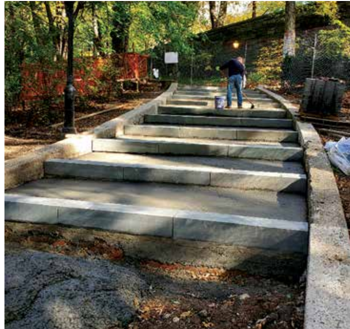
The work in progress at the 114th Street step ramp.
