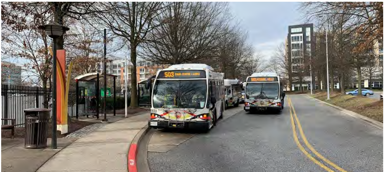
Figure 2-4: Columbia Mall Transit Center
