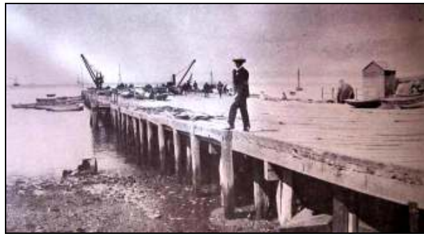
Plate 11: Photograph of the wooden jetty (Central jetty) at the end of Adderley Street c1902 (Picard 1969:118). The central jetty was constructed in the 1850's and became the central hub of harbour activities. In 1907 the jetty was extended to create a central pier and promenade. The pier was demolished in 1938 to make way for the Foreshore Reclamation Scheme (Patrick et al 2010).
