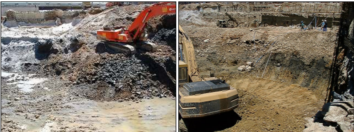
Plates 23 & 24: At left two types of fill consisting of the lower rock rich deposits (from the base of Duncan Dock?) and sea/dune sand above. A thick dark layer in the photograph at right, was interpreted as the old seabed, upon which was a build up of organic debris and coal residue (Photographs: ACO Associates archive).
