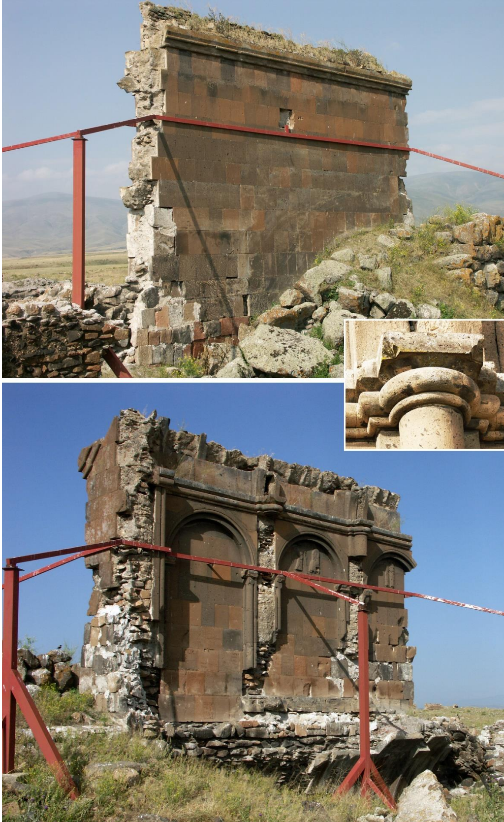
Fig. 15. Ani. “Georgian church”. Present state of the monument. The northern wall seen from the northeast and from the southwest. Detail of the capital surmounting the eastern half-column of the northern wall (Photos: Patrick Donabédian)
