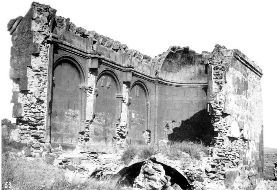
Fig. 13. Ani. “Georgian church”. Plan after KARAPETYAN, Ani 1050 , 211, fig. 554 (measurement by T. Toramanyan, early 20 th c.). Southwest view. Photo T. Toramanyan (early 20 th c.). Archives of the History Museum of Armenia, Yerevan.
