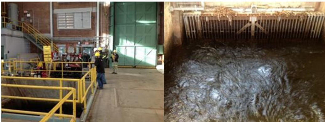
Figure 3-1: Water intake at the central Shawinigan 2.
